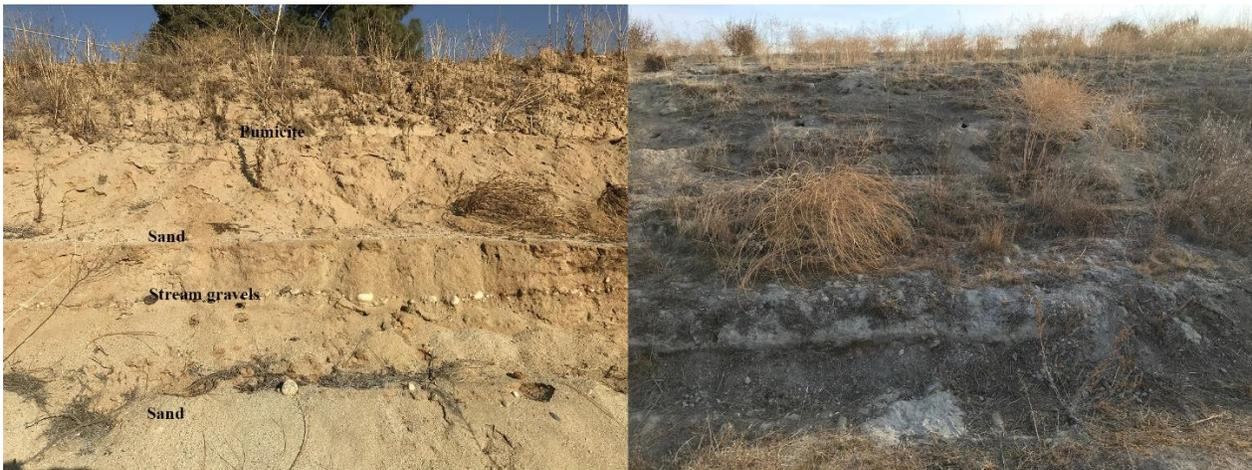
Figure 13. 8 ft road cut on the eastern half of the Copper River Development showing layers of alluvium deposits.
