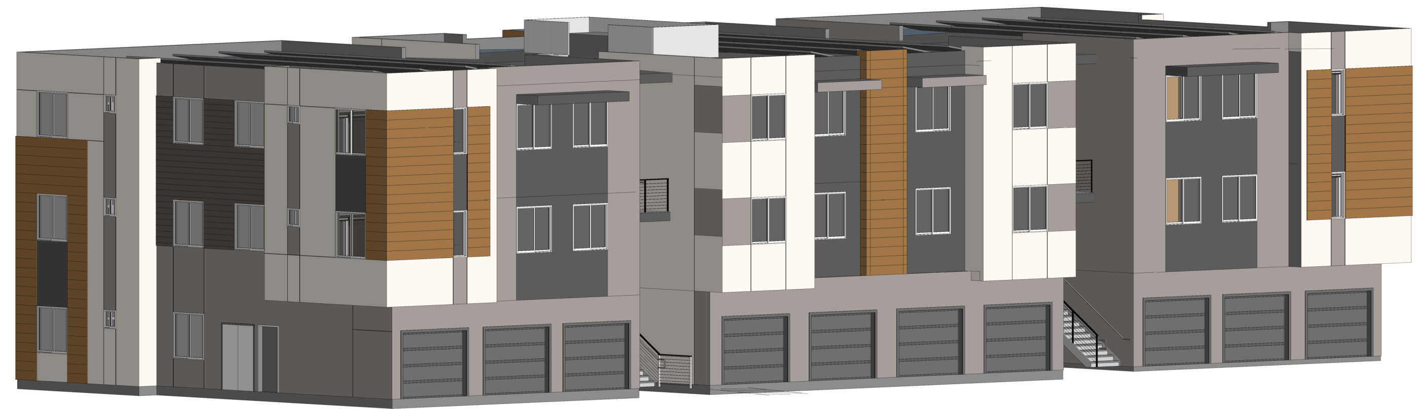
3. NORTH / WEST - VIEW
