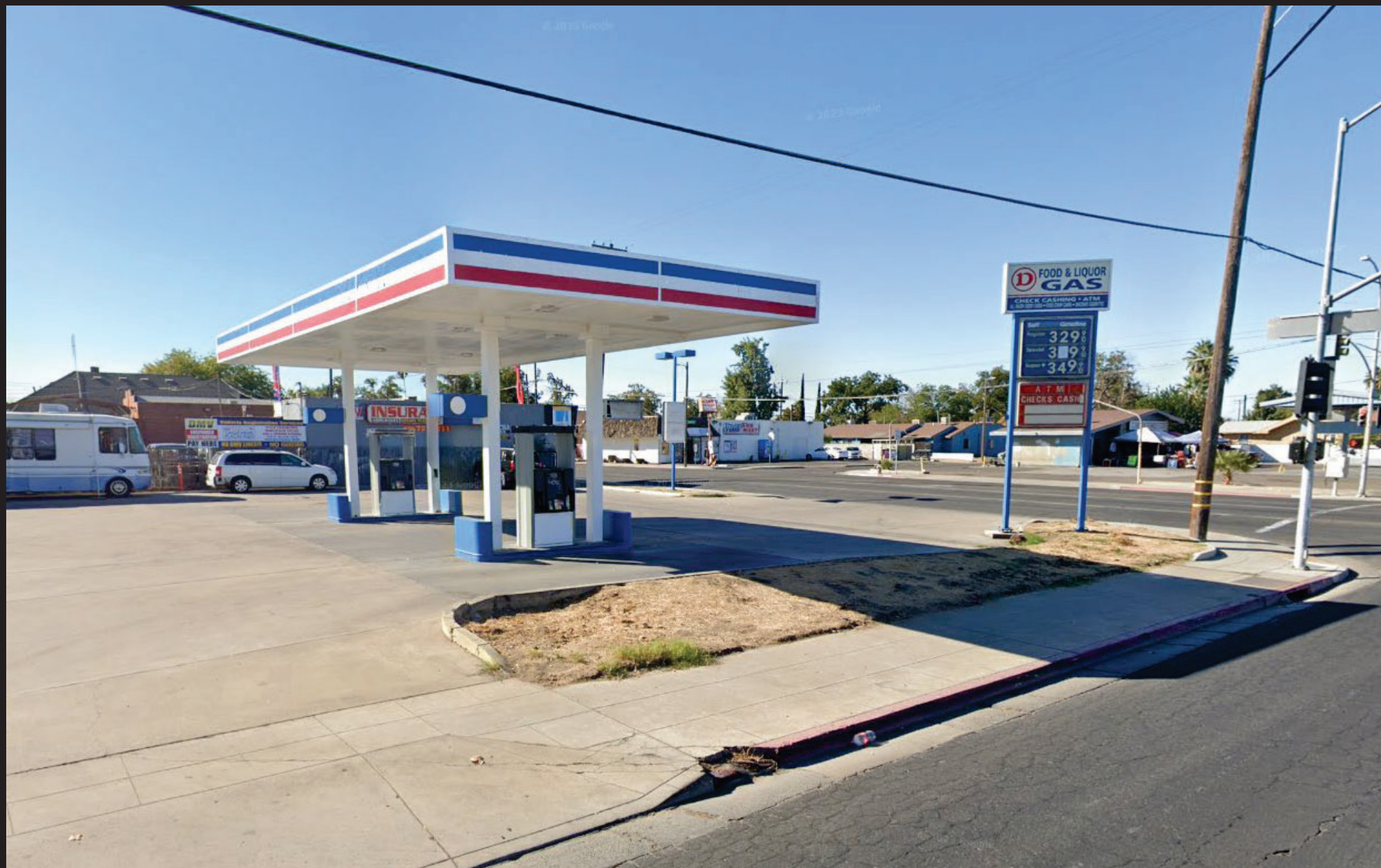
Canopy & Gas Pumps – 2520 E. Olive Ave.
