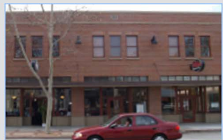
The windows of this mixed-use building are composed according to a logical order. The second floor windows are grouped in threes and centered above the ground floor storefront doors and windows.
