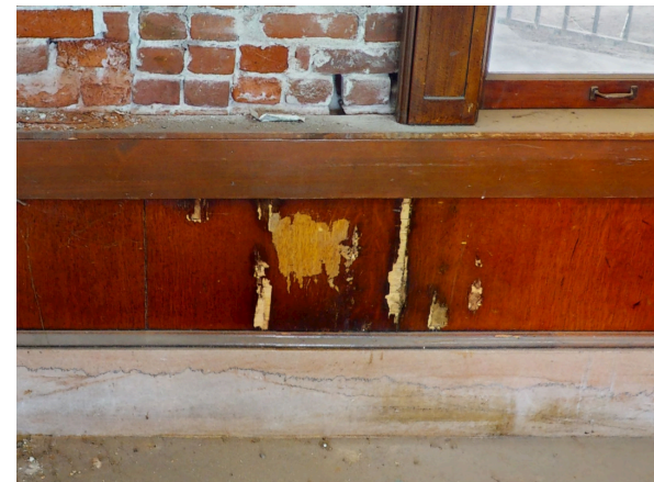
Example of existing damage at wainscoting
