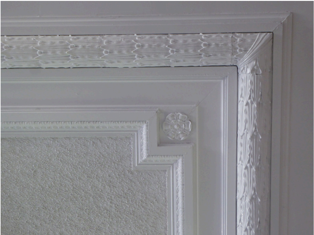
Existing plaster ceiling ornament with wood trim elements and non-historic acoustic texture
