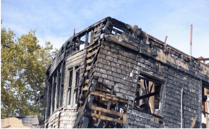
South-east corner as viewed from east neighboring property.
