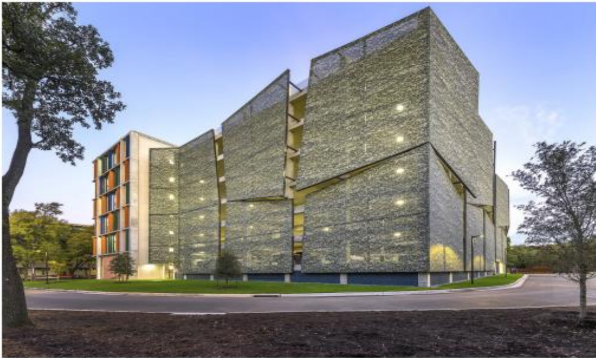
Rice University Cambridg Office Garage, Houston, TX • Tensile Mesh Facade, Custom Printed with Leaf Pattern Image
