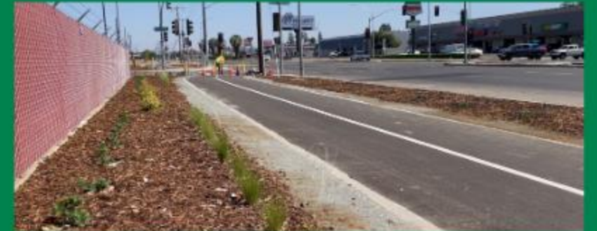
Approximately 10.63 miles of Class I trail facilities were added to the trail network.
