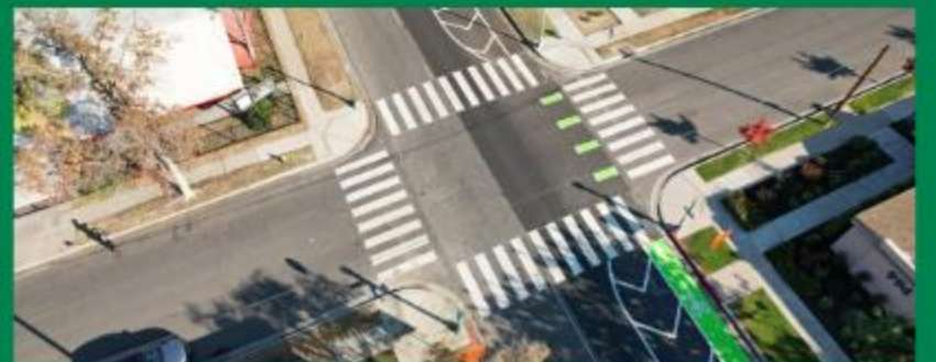
30 new crosswalks, 375 ADA ramps, and 237 streetlights were installed throughout the City.
