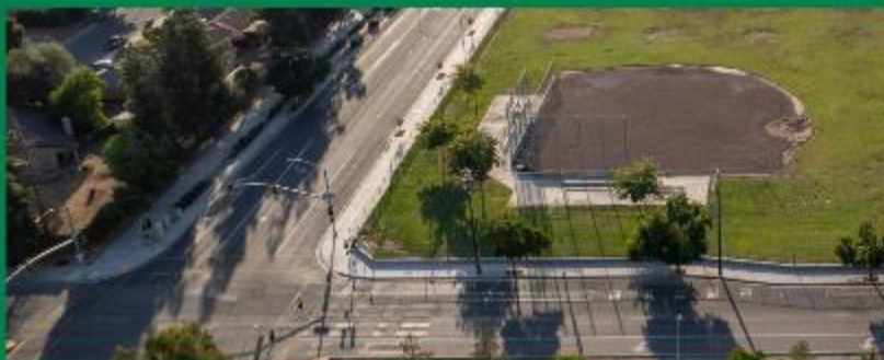
Over 11 miles of sidewalks constructed and 7.5 miles of existing sidewalks repaired.
