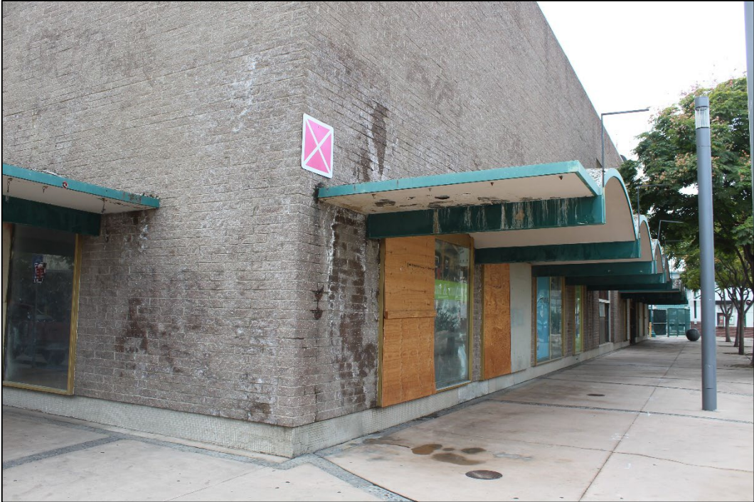
Figure 7. Detail of north corner of 887 Fulton Street, facing south (Stantec, 2025).
