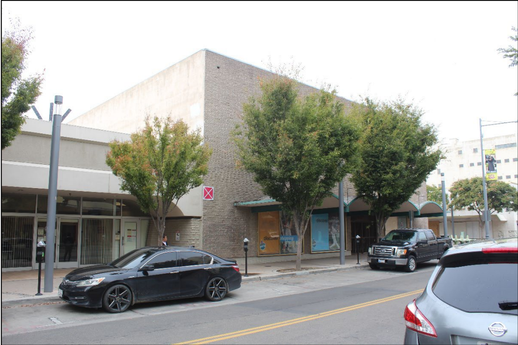
Figure 3. Fulton Street façade of 887 Fulton Street, facing northwest (Stantec, 2025).
