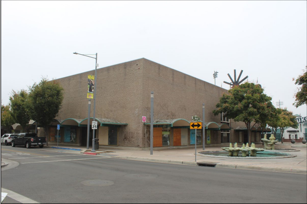
Figure 2. Overview of 887 Fulton Street from Fulton Street, facing south (Stantec, 2025).
