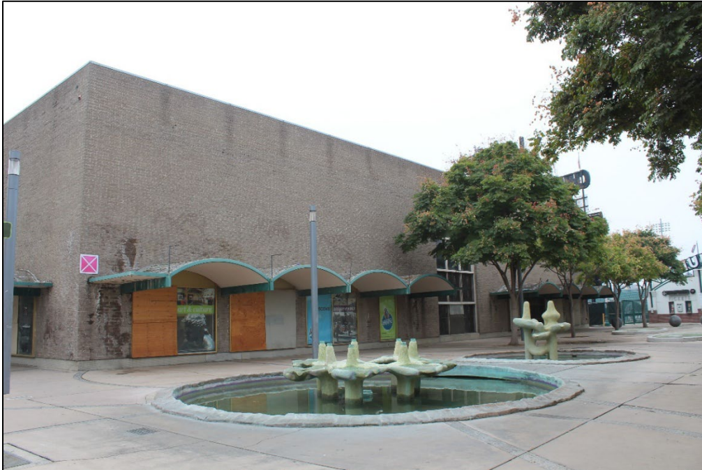
Figure 4. North façade of 887 Fulton Street, facing south (Stantec, 2025).
