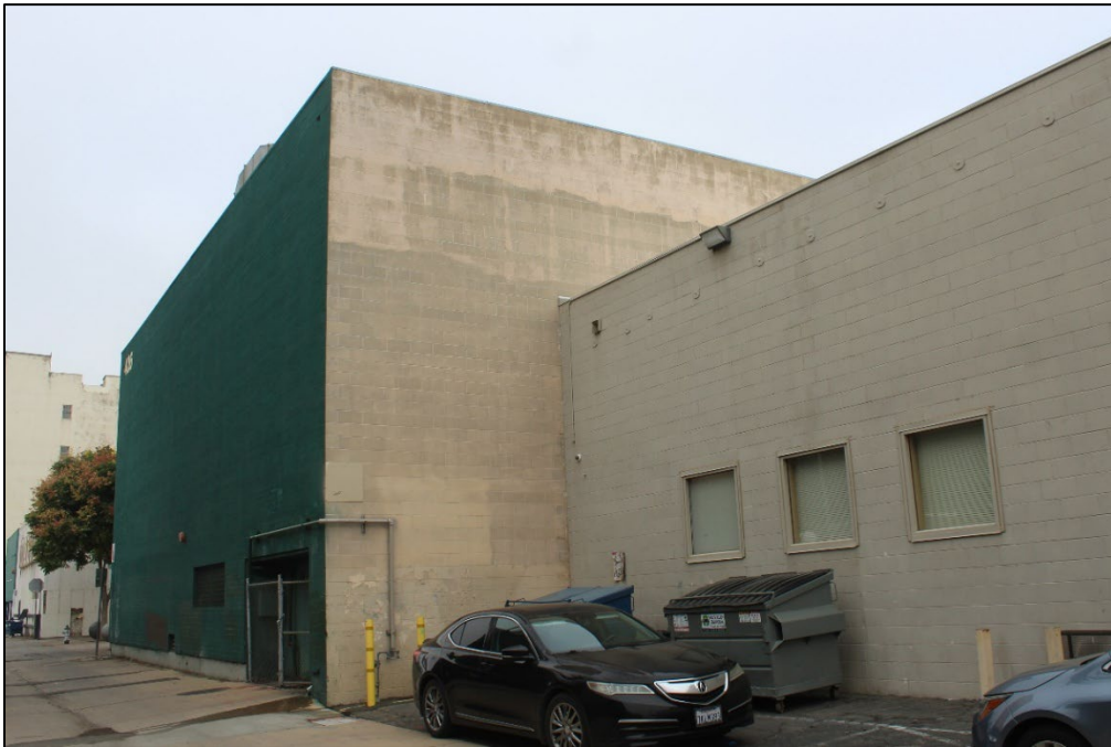
Figure 11. Rear of 887 Fulton Street on Homerun Alley, at left, facing north (Stantec, 2025).
