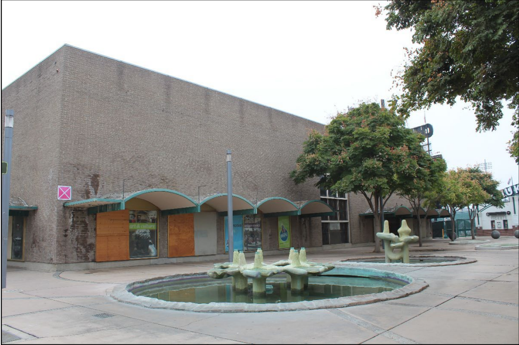
Figure 6. North façade of 887 Fulton Street, facing south (Stantec, 2025).
