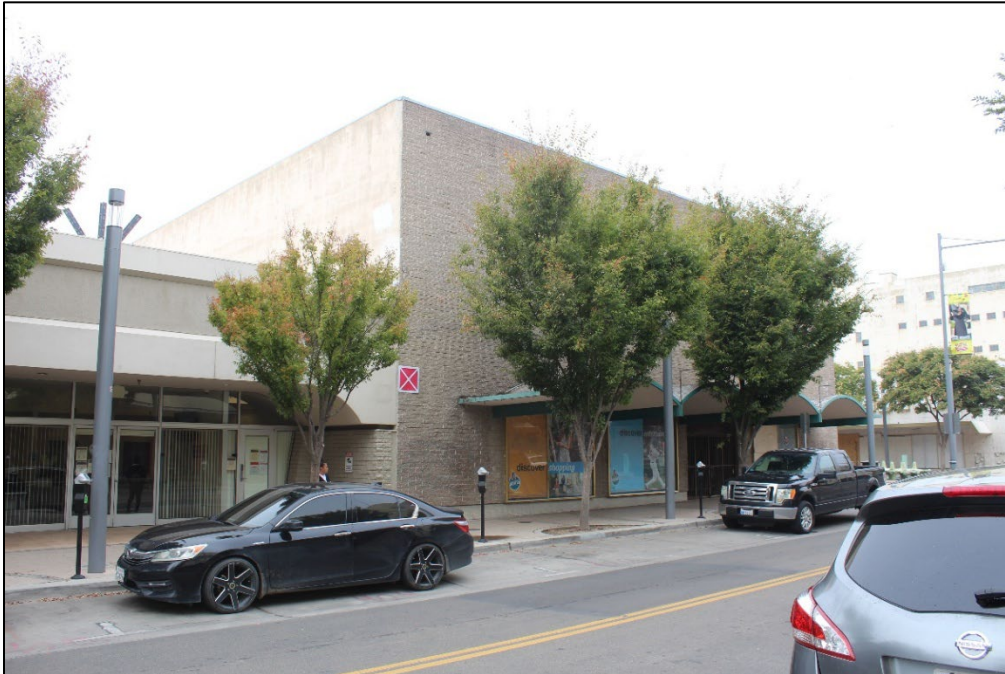
Figure 1. Fulton Street façade of 887 Fulton Street, facing northwest (Stantec, 2025).
