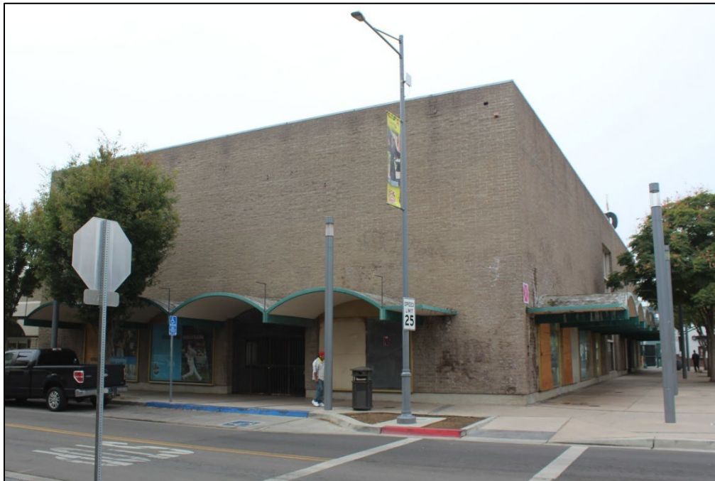
Figure 2. Fulton Street façade of 887 Fulton Street, facing southwest (Stantec, 2025).
