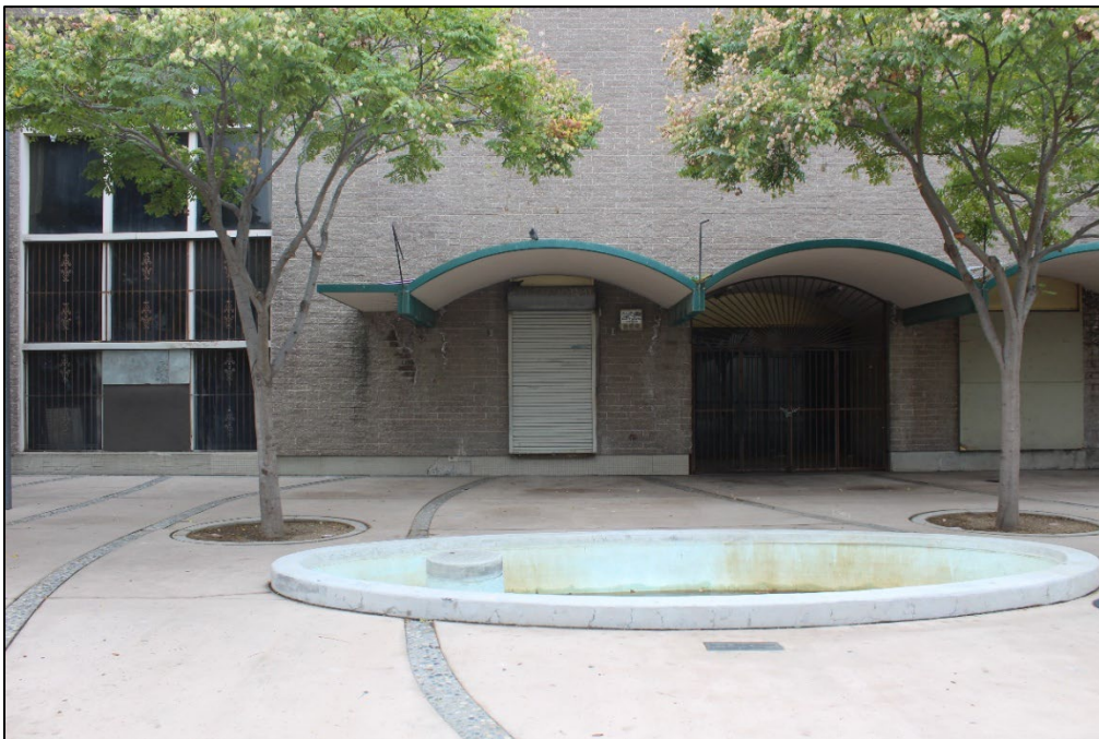
Figure 7. The north façade entrance to the building, at right, facing southeast (Stantec, 2025).
