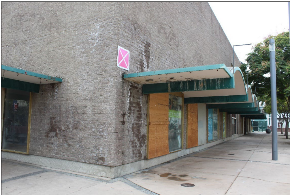
Figure 5. Detail of north corner of 887 Fulton Street, facing south (Stantec, 2025).
