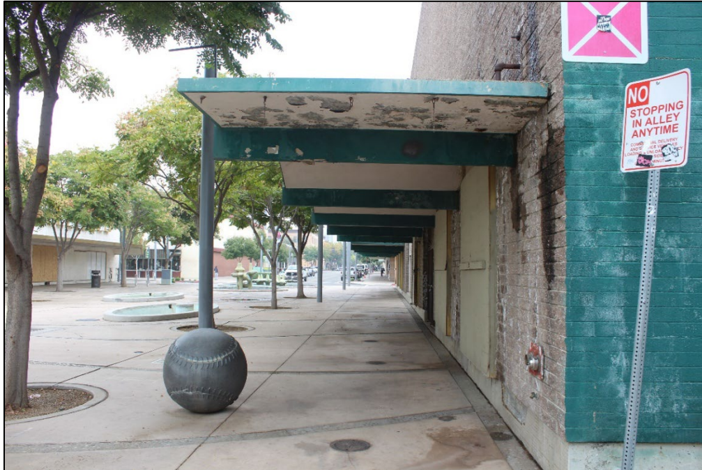
Figure 8. Detail of the cantilevered concrete canopy on the north façade of the building, facing northeast (Stantec, 2025).
