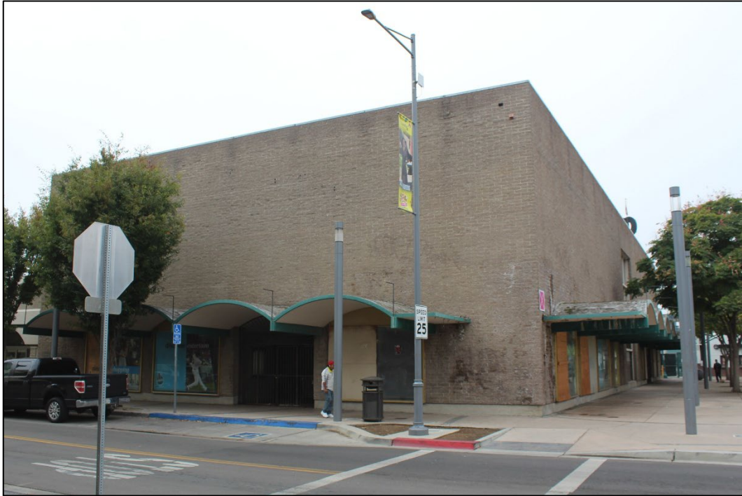
Figure 4. Fulton Street façade of 887 Fulton Street, facing southwest (Stantec, 2025).
