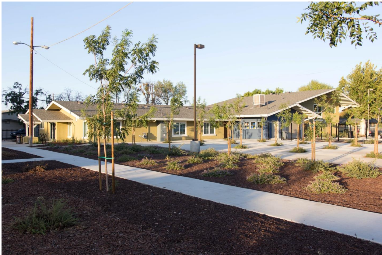
Cedar Courts, completed in 2015
