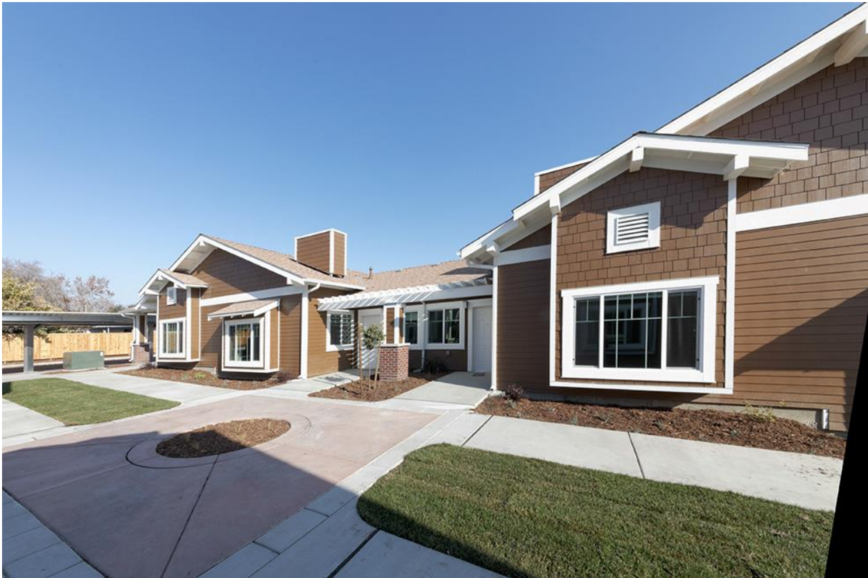
Bridges at Florence, completed in 2014
