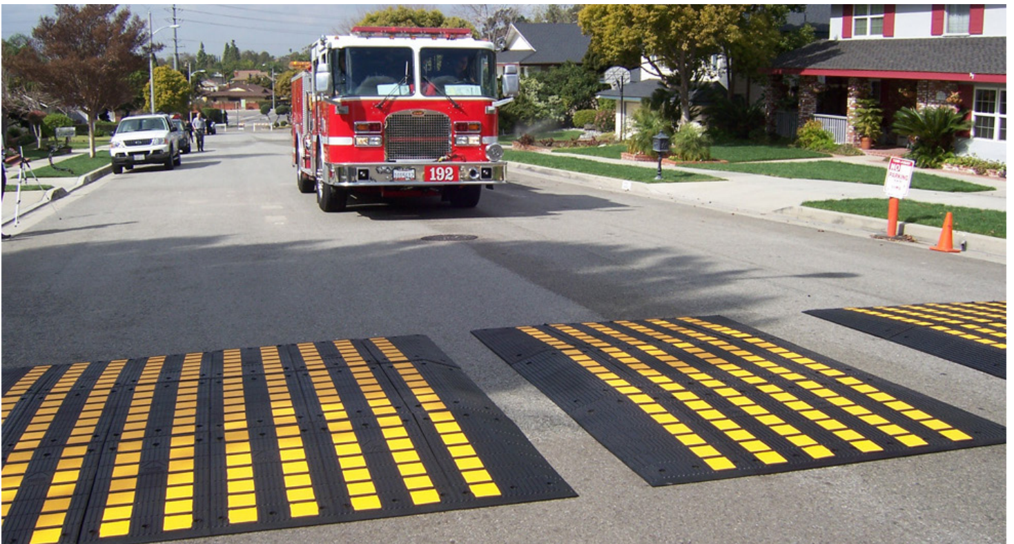
Figure 4.6: Speed Hump (source: NACTO https://nacto.org/publication/urban-street-design-guide/street-design-elements/vertical-speed-control-elements/speed-cushion/ )
