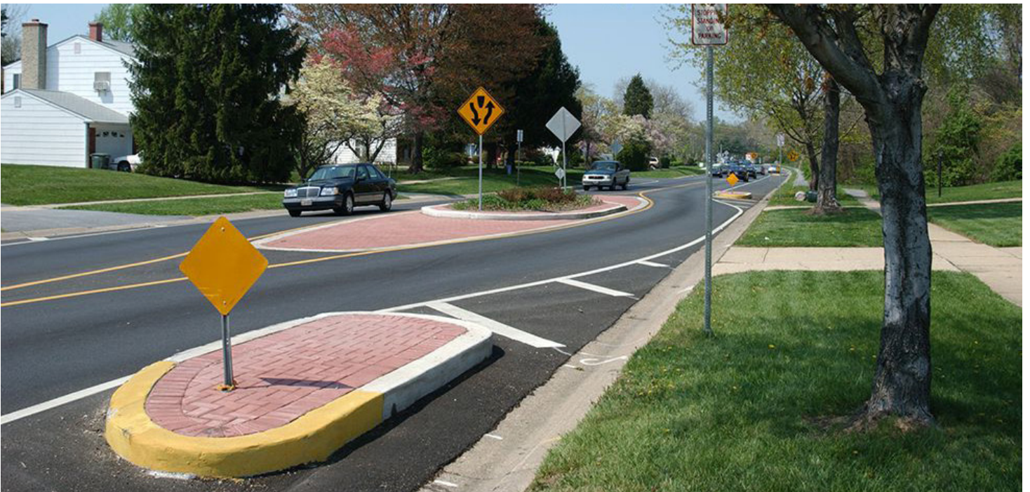
Figure 4.8: Chicane (source: NACTO https://nacto.org/publication/urban-street-design-guide/street-design-elements/curb-extensions/chicane/ )
