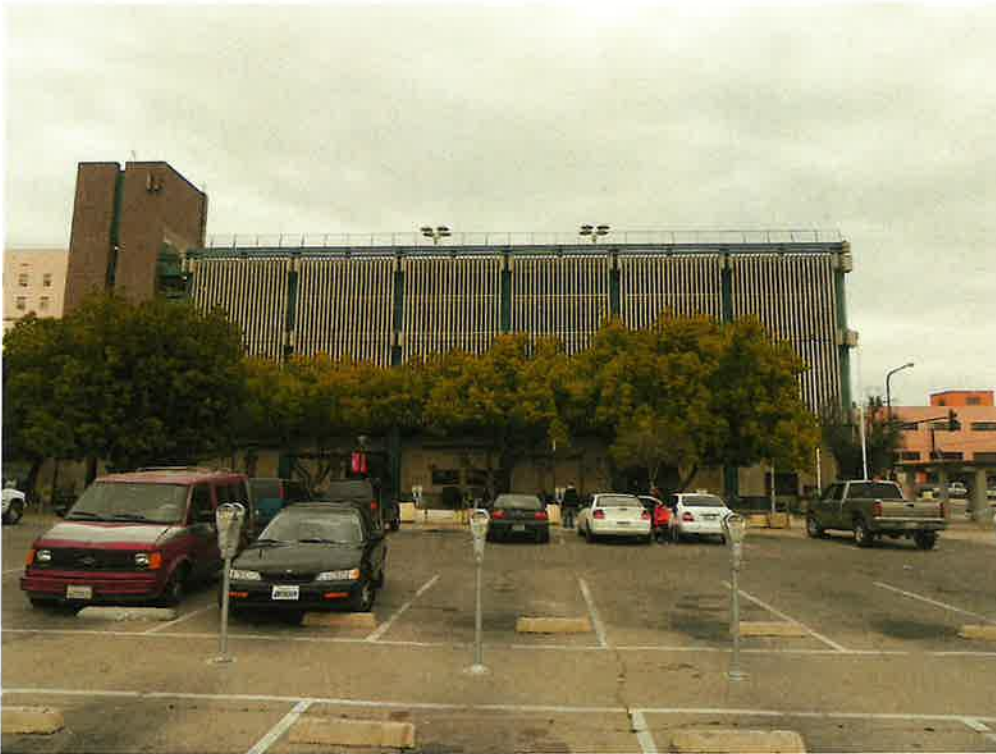
860 Fulton Mall, Southwest elevation, March 1, 2011.
