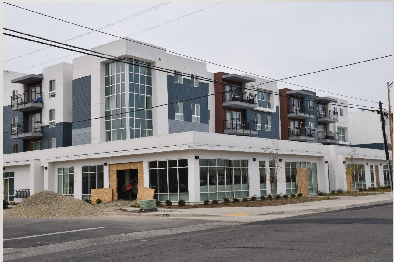
The Link at Blackstone & McKinley - 87 MF units
