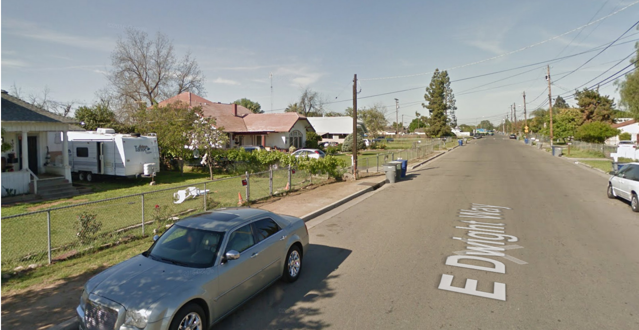
Example of missing and incomplete sidewalk segment along East Dwight Way
