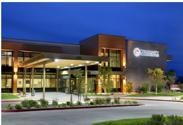
Community health center. Photo credit. FCI Constructors
