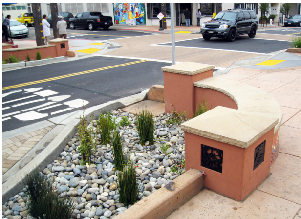
High visibility crossing and decorate bulbout with rain gardens. Photo credit: VMWP
