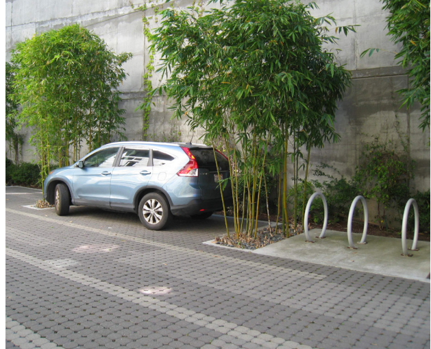
Permeable parking lot paving
