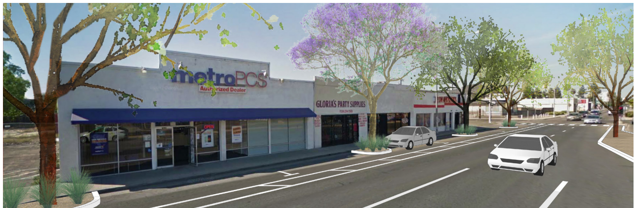
The first step in the transformation of Cesar Chavez Blvd should involve streetscape improvements that provide an inviting public realm, such as: restriping lanes to add on-street parking with bulb-out planters to shade the sidewalk and adding a buffered bike lane. Now, Cesar Chavez Blvd will provide a multimodal environment.
