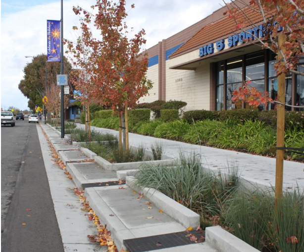
Rain garden in planter strip
