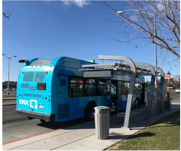
New BRT Station on Cesar Chavez Blvd
