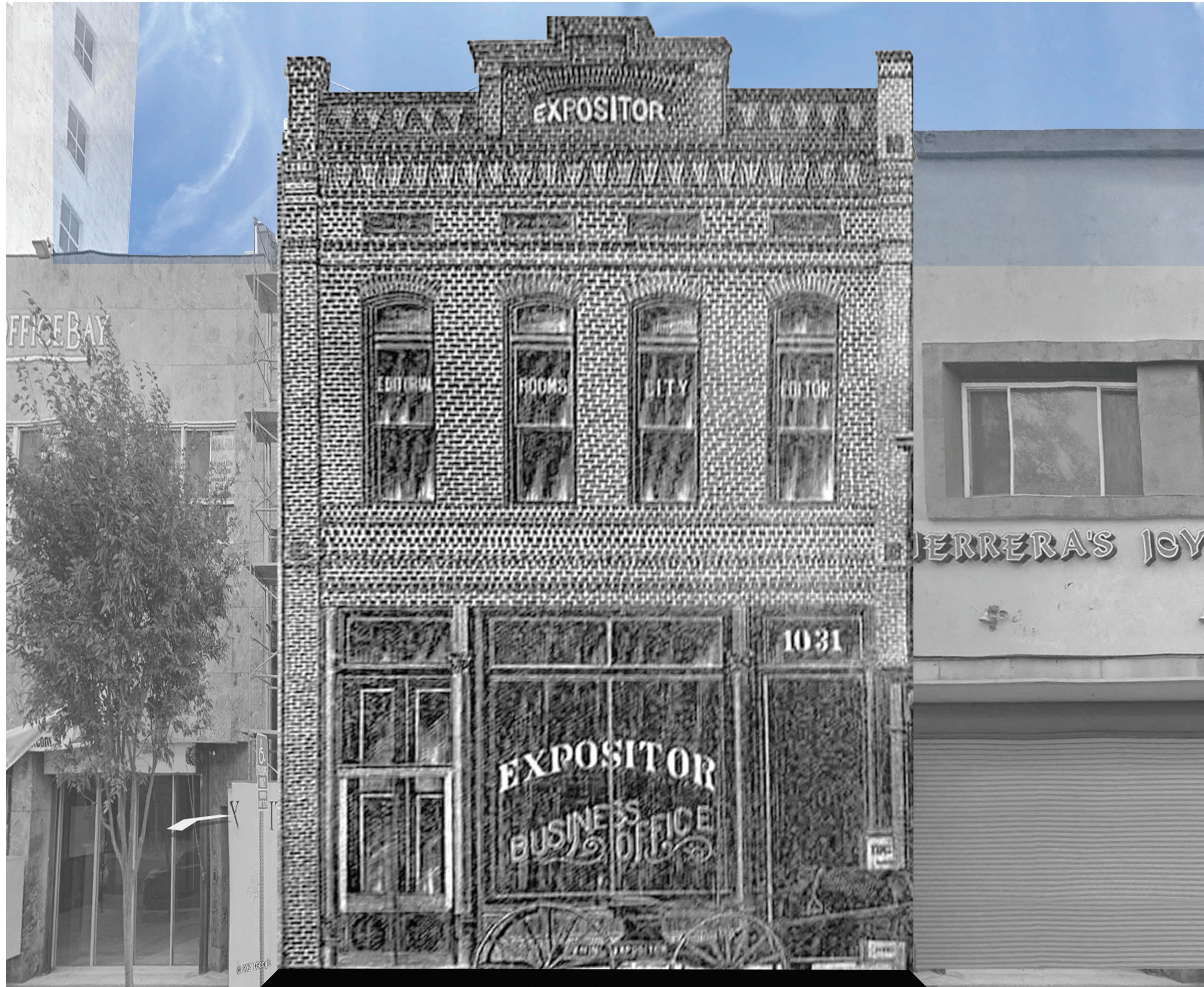
Archival Facade Image
