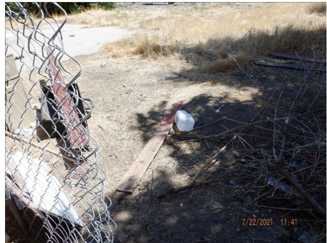
Date: 7/22/2021 11:41:20 AM Interior of backyard where temp fence panel has been cut at alley. TDS
