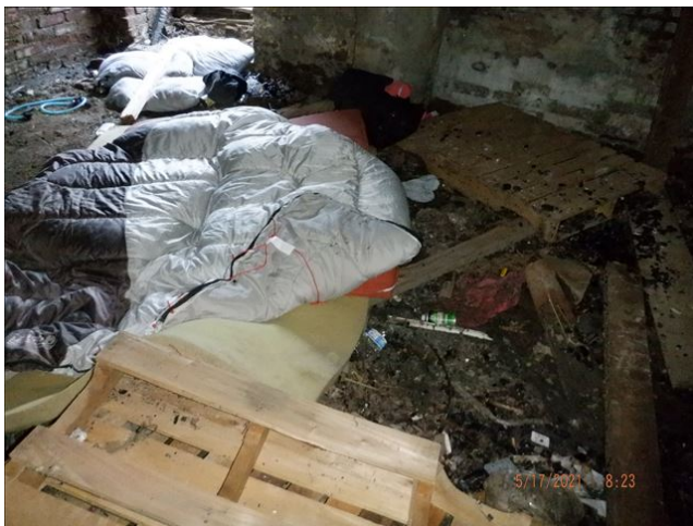
Date: 5/17/2021 8:23:18 AM Sleeping arrangements in basement appear new and show no signs of fire damage or debris. TDS
