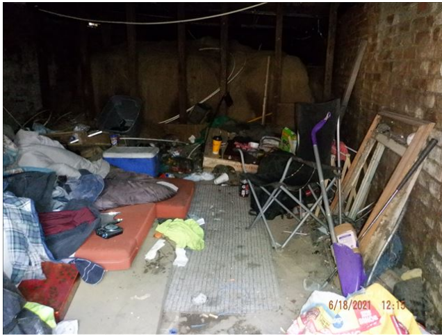
Date: 6/18/2021 12:15:40 PM Indications of person(s) living in basement of multiunit dwelling. Recovered stripped electrical wire, razor blade, metal detector and hypodermic needles from basement. TDS
