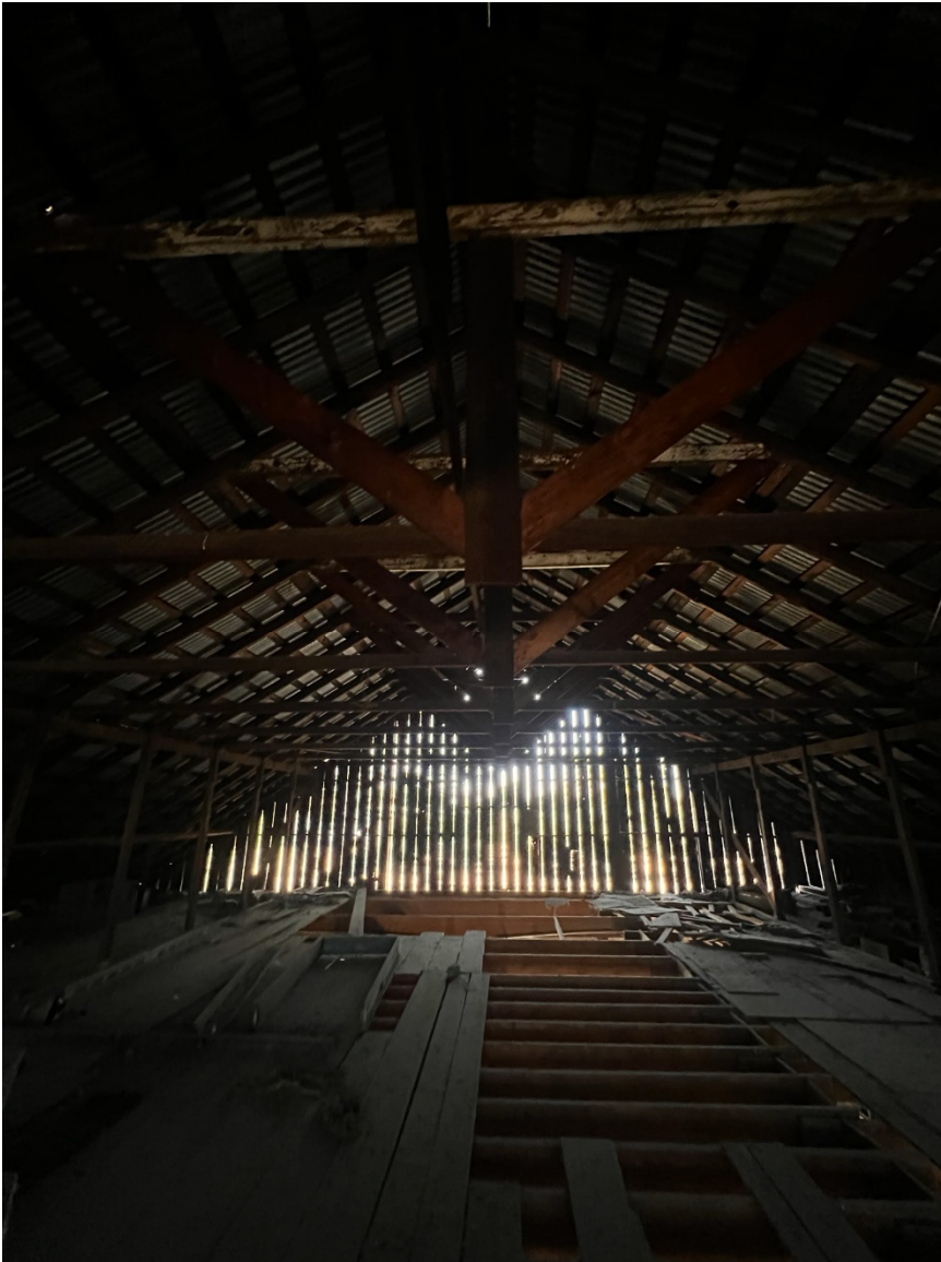
Photograph No. 2 Field built trusses
