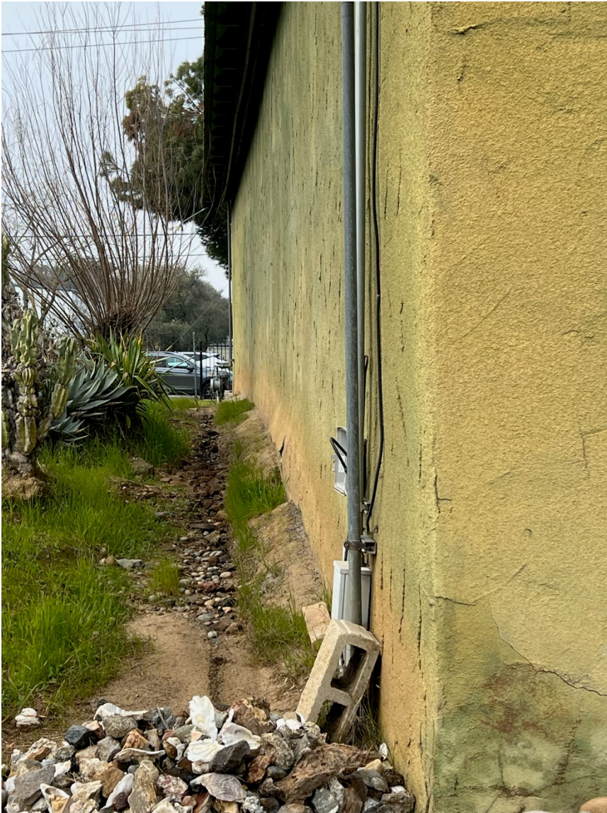
Photograph No. 4 Adobe walls covered by plaster
