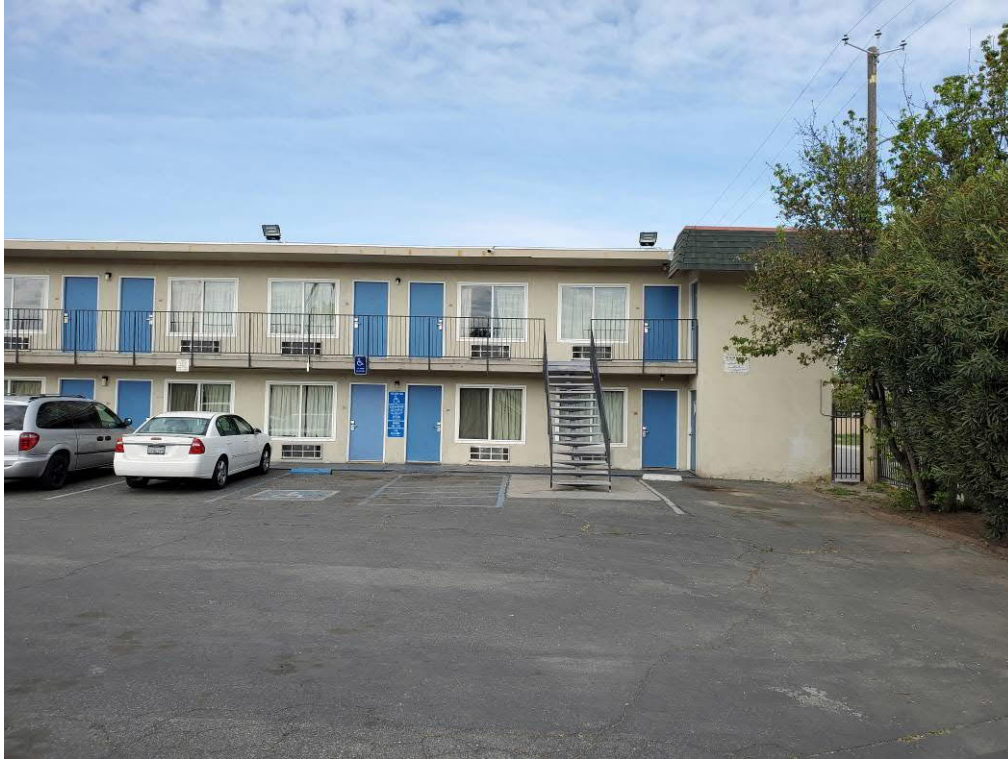
Photo 3: Central northern portion of subject site, facing west. Western two-story motel building in background.
