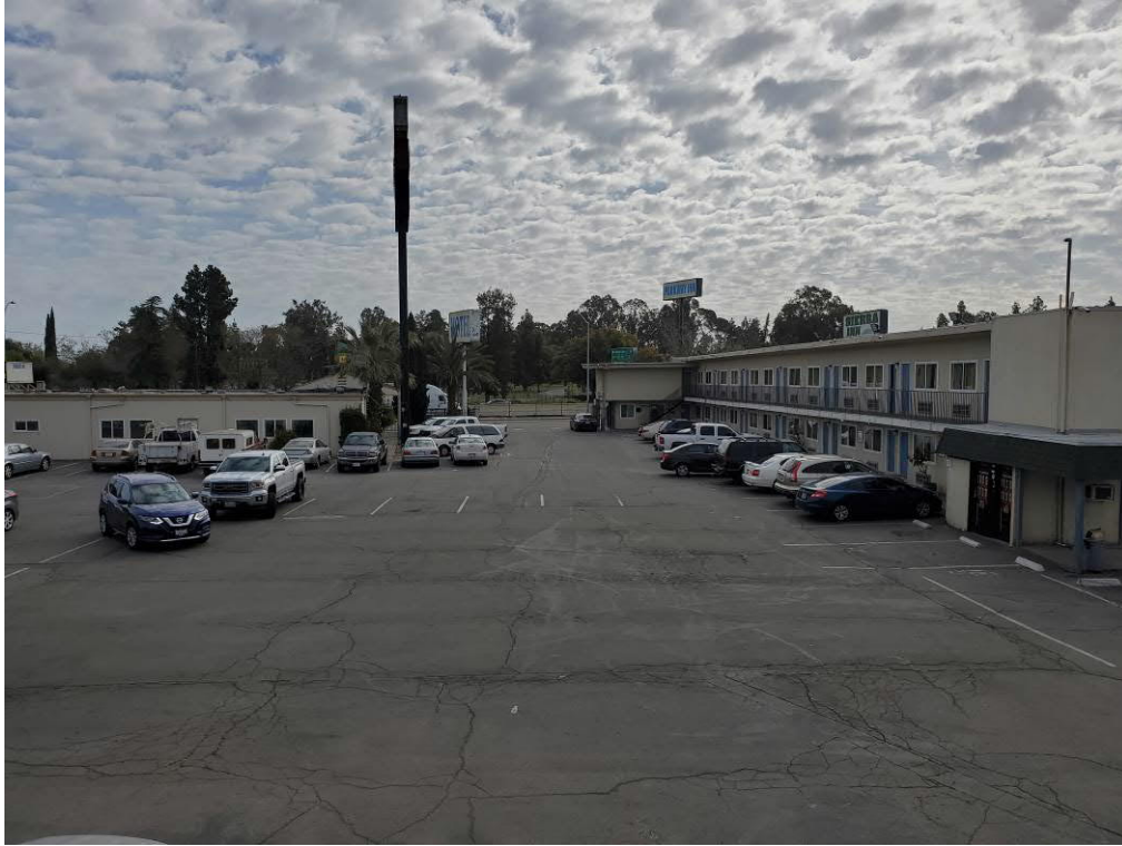
Photo 1: Central western portion of subject site, facing east. One-story former restaurant building on the left, eastern two-story motel building on the right.
