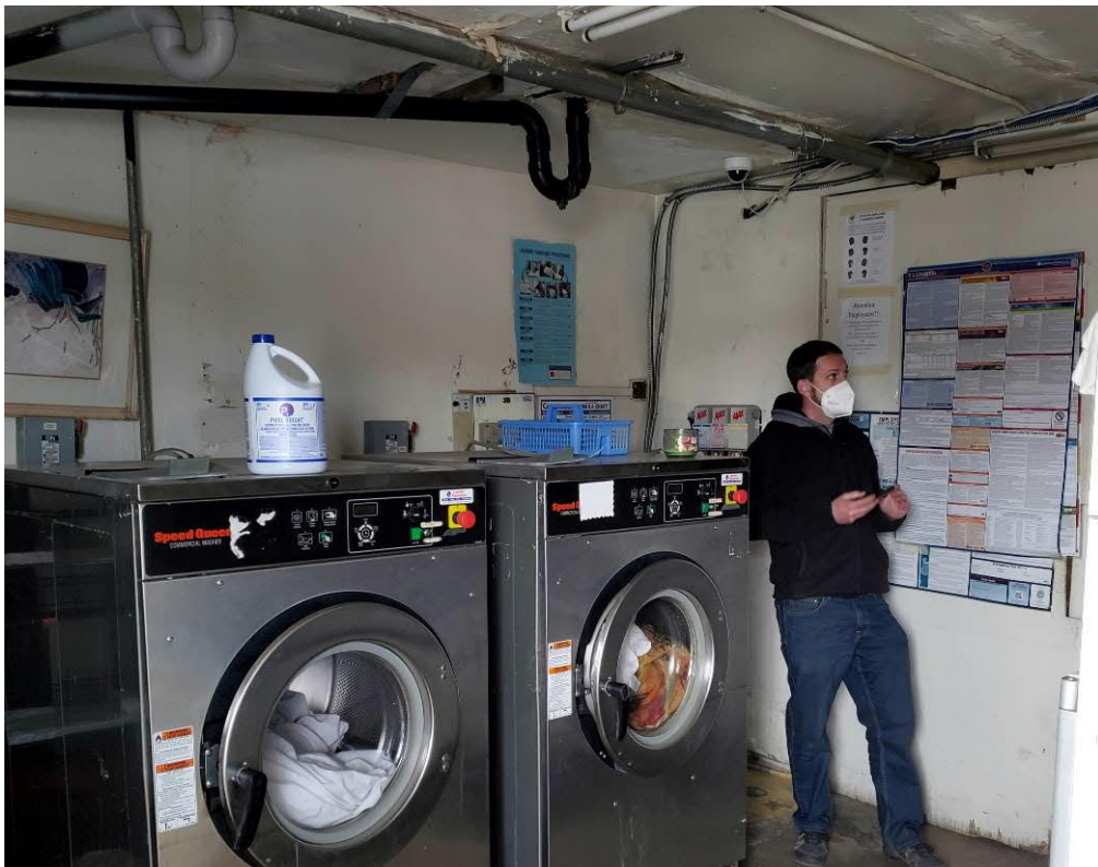
Photo 9: Western portion of subject site, first floor. Motel laundry.
