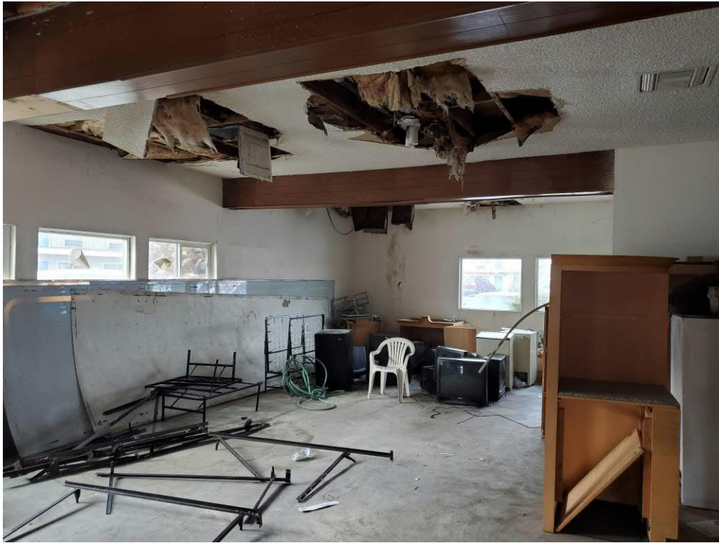
Photo 5: Interior of vacant one-story building in northeastern corner of subject site.
