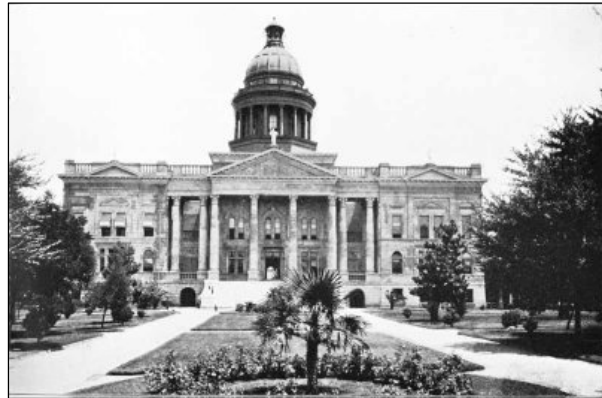
Fresno County Courthouse (demolished) Fresno Historical Society Archives
