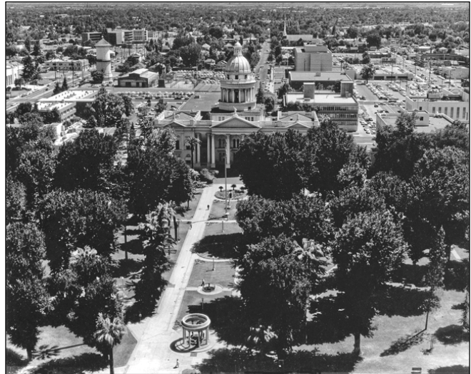
County Courthouse and Courthouse Square 1962 Image courtesy of Lance & Cromwell.
