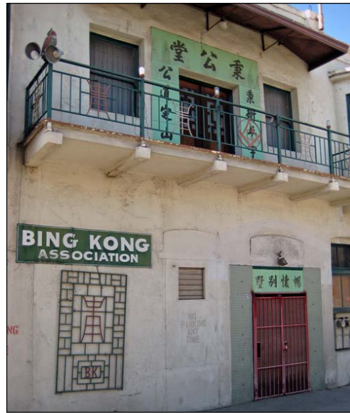
Bing Kong Association Building (1900)
