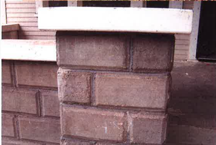
215 N. Clark Street looking northwest; rusticated concrete brick piers.
