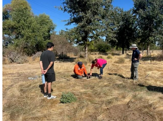
Native Garden Irrigation Restoration
