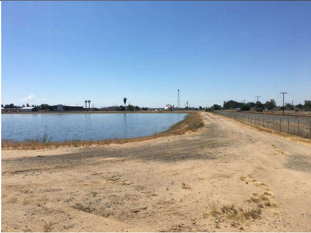
Image 5: Overview of 0.33 miles east of Brawley Avenue showing east end of water retention facility, looking west.
