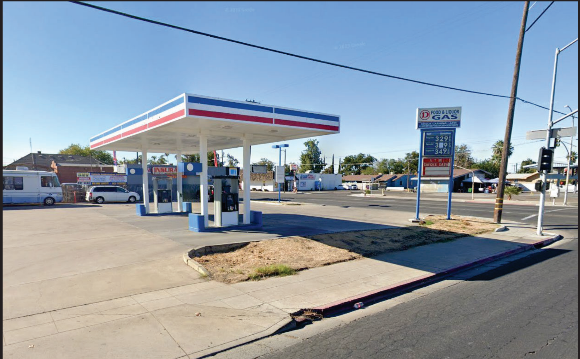
Canopy & Gas Pumps – 2520 E. Olive Ave.
