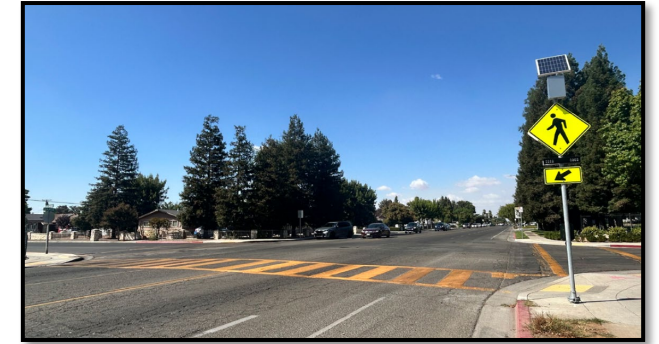
Rectangular Rapid Flashing Beacons
