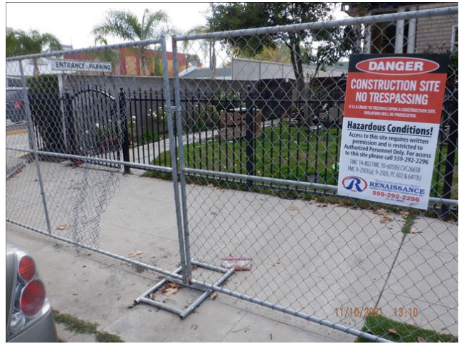
Date: 11/10/2021 1:10:53 PM Opening cut in temporary fence panel on north side of property on L Street side. TDS
