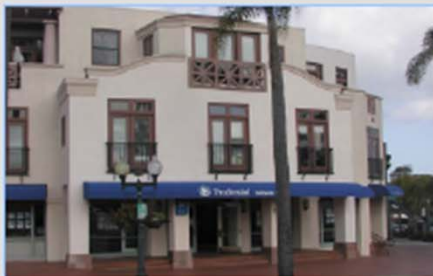
A mixed-use building clad in plaster. The moldings and column bases are constructed of durable materials (precast concrete and tile, respectively).
