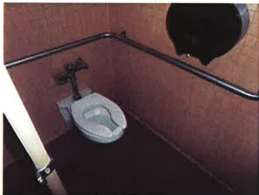
Photo #52: Toilet stall at Building B is too narrow
