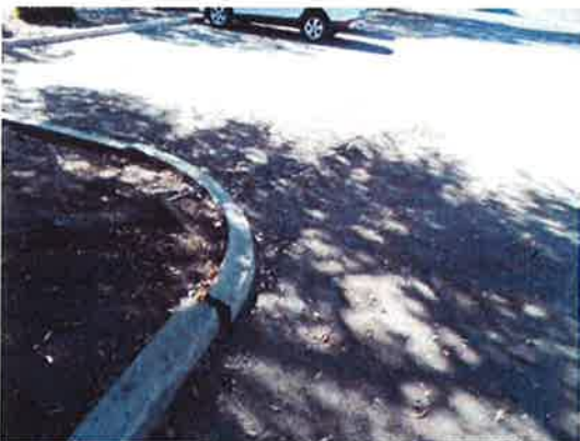
Photo #9: Cracked curbing
