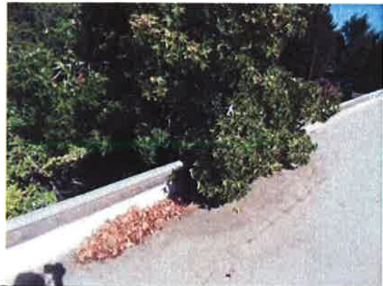
Photo #8: Overgrown trees on roof
