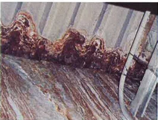
Photo #17: Leak at metal deck Building A
