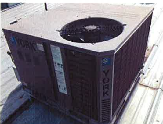
Photo #65: Typical newer package unit
