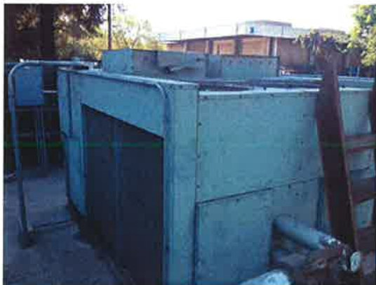
Photo #55: Air Cooled chiller for Building A
