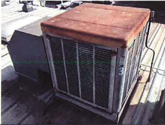
Photo #61: Evaporative cooler with fan duct at Building F
