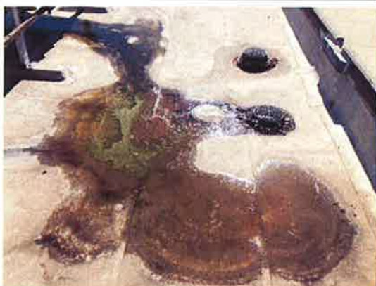
Photo #60: Condensate water leaking and ponding at Building B
