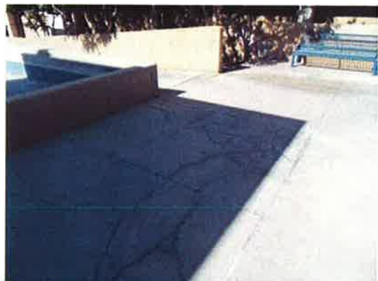
Photo #16: Cracking near Building A fountain causing leak below
