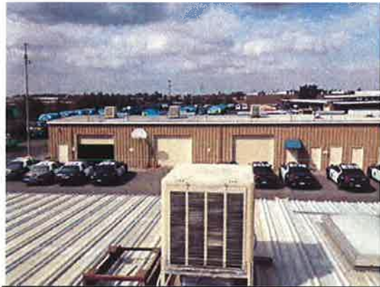
Photo #62: Evaporative cooler at Building X
