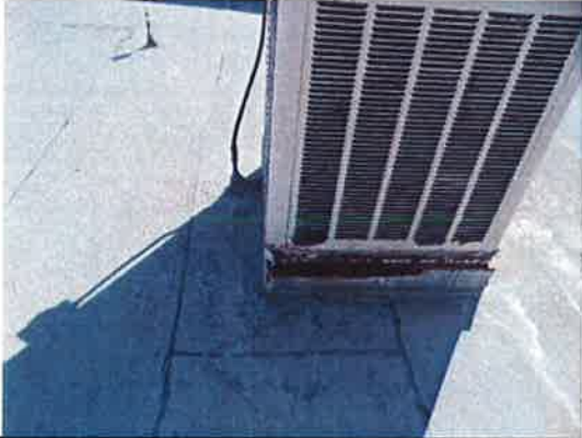
Photo #25: Roof at Building T with rust at evaporative cooler connection
