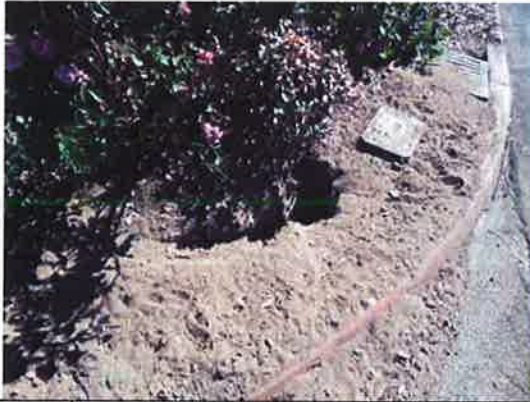
Photo #7: Isolated irrigation leak
