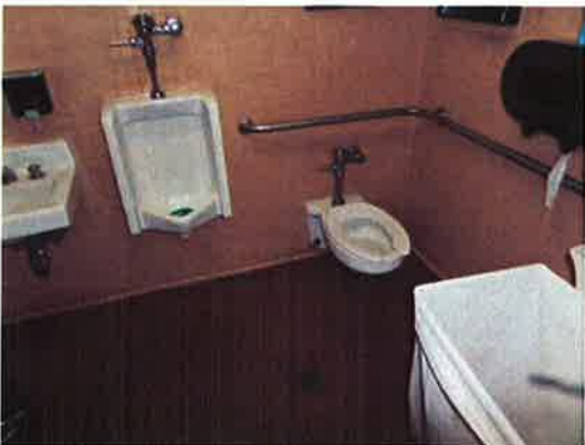
Photo #47: Restroom at Building E requires pipe wrapping and lever handles at lavatory
