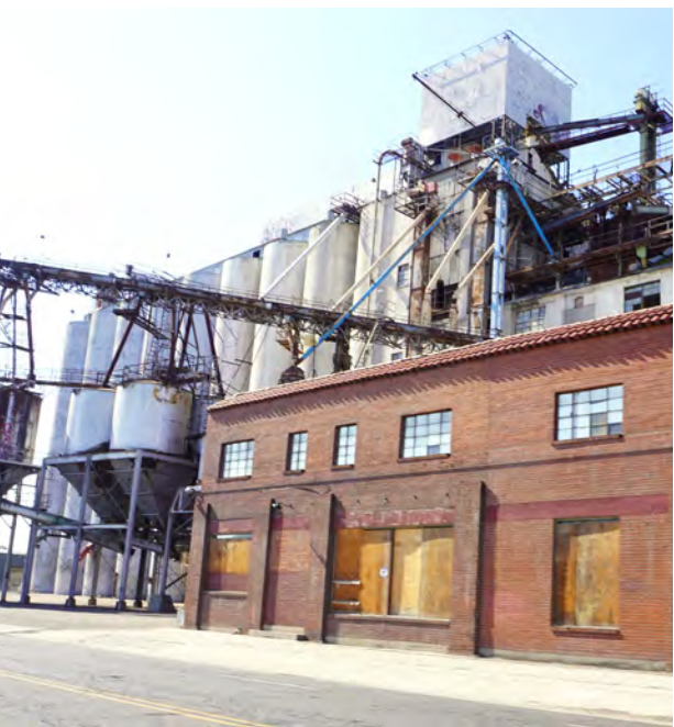
Grain silos in southwest corner of Tower District
