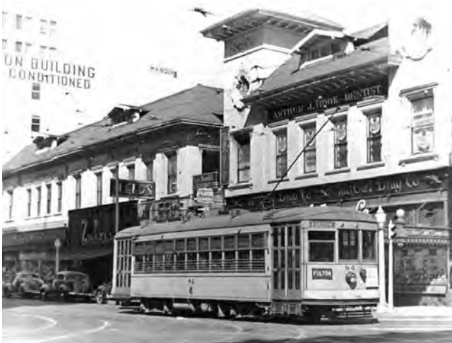
Historic streetcar running along Fulton Street Source: Interurbans Publications
