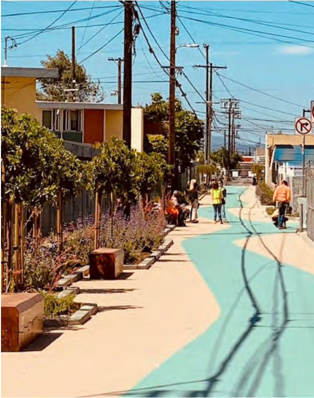
Using alleys to enhance the bike and pedestrian network, access ADUs and create greenways.
