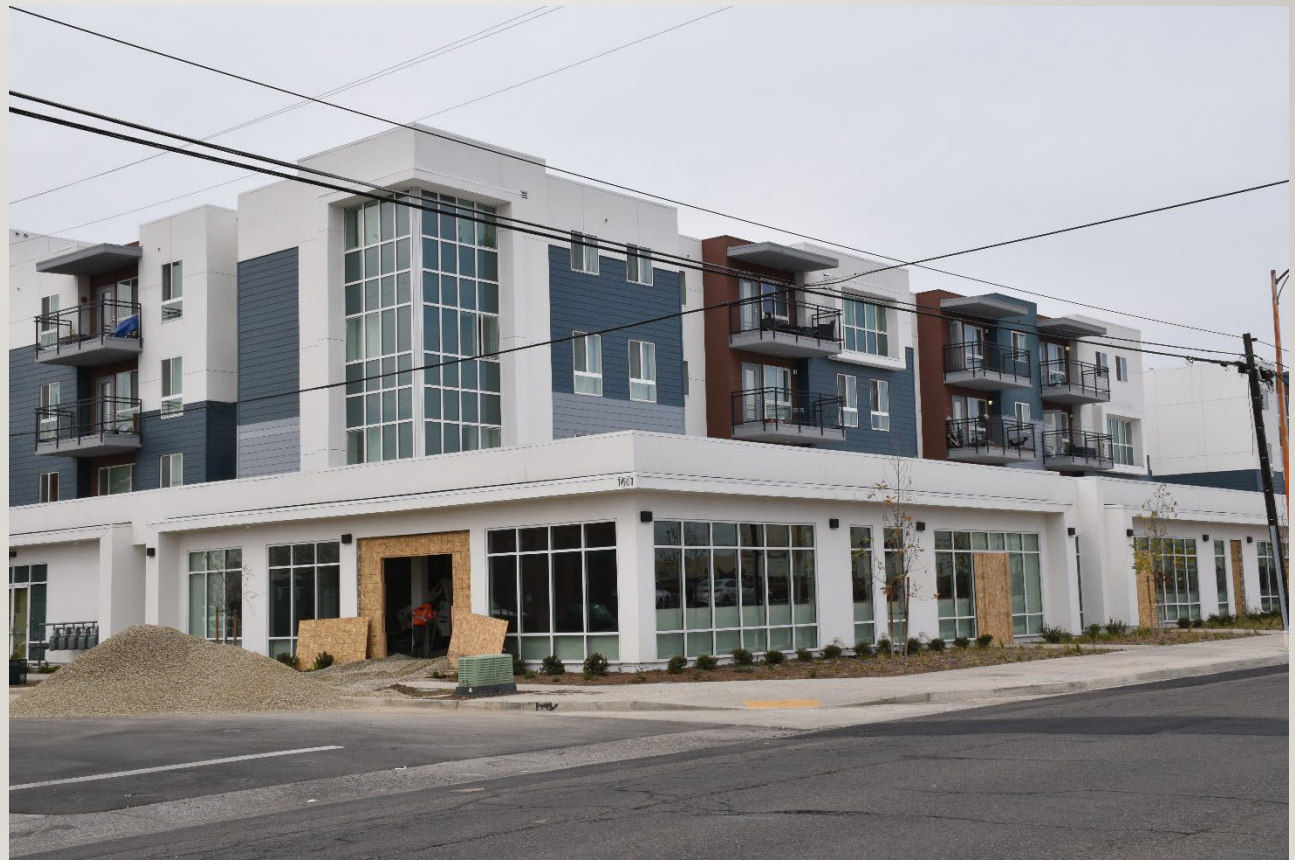
The Link at Blackstone & McKinley - 87 MF units
