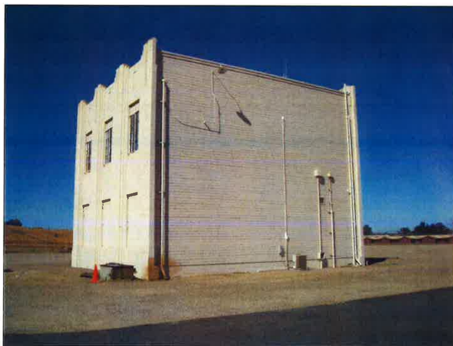
South and east elevations of Feature I, the Control Building (August 2008).
