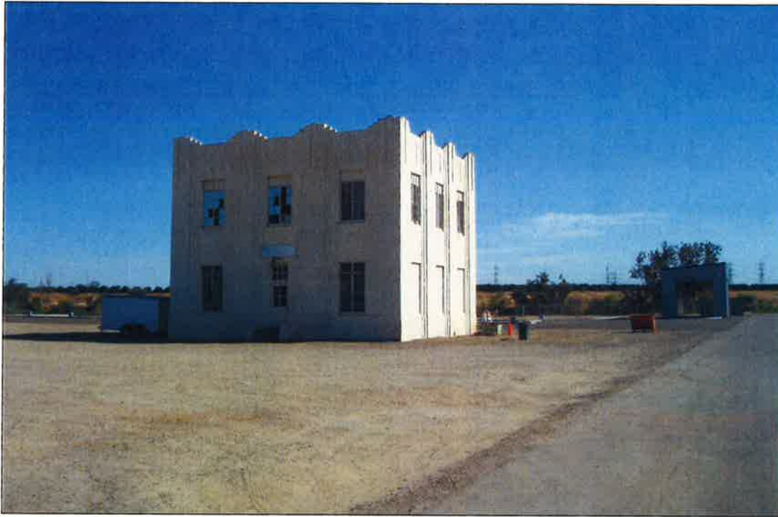
Figure 4-4 West and south façades of the Control Building (Applied EarthWorks, August 2008).
