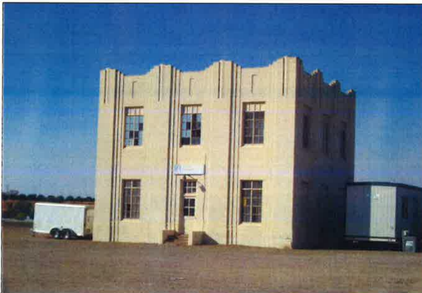
View looking northeast at west elevation of Feature I, the Control Building (August 2008).
