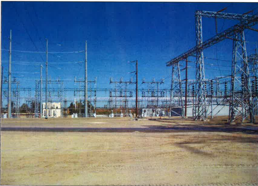
Figure 4-3 View from the same angle illustrating the changes at the substation in the last 77 years (Applied EarthWorks, August 2008).
