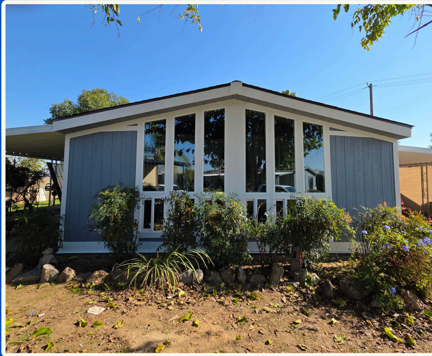
Mobile Home Repair
