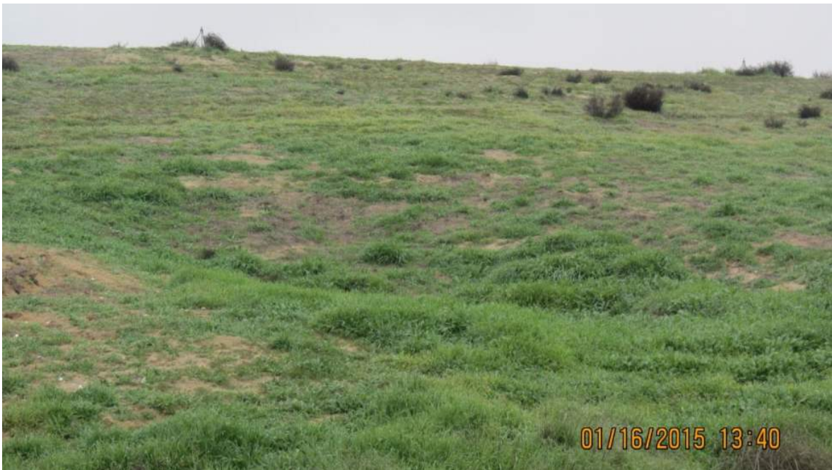
Photo 15: Subsidence on Eastern Face of Landfill
