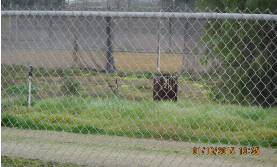
Photo 12: Detention Pond Standpipe Leading to Paintball Area
