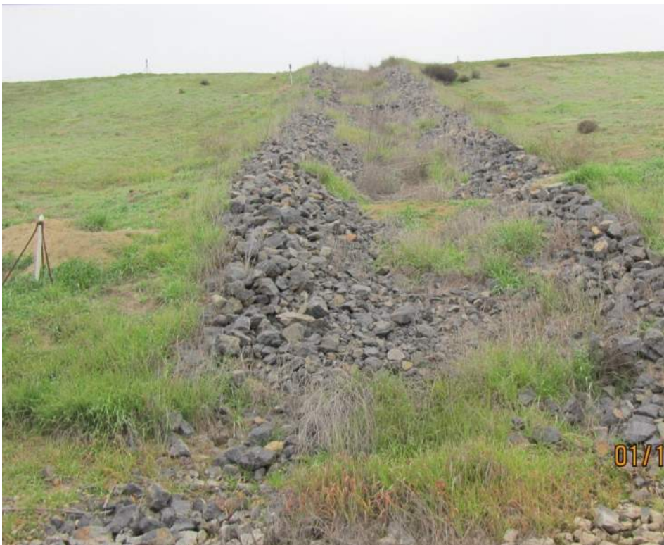
Photo 13: Surface Water Drainage from Top of the Landfill
