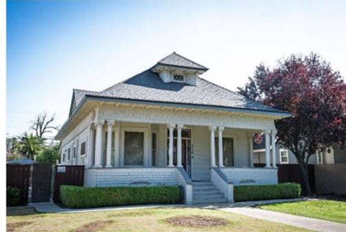
3) Historic Preservation Program (Roof Replacement)
