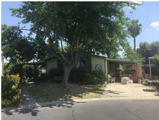
2) Mobile Home & Repair and Replacement Programs Before
