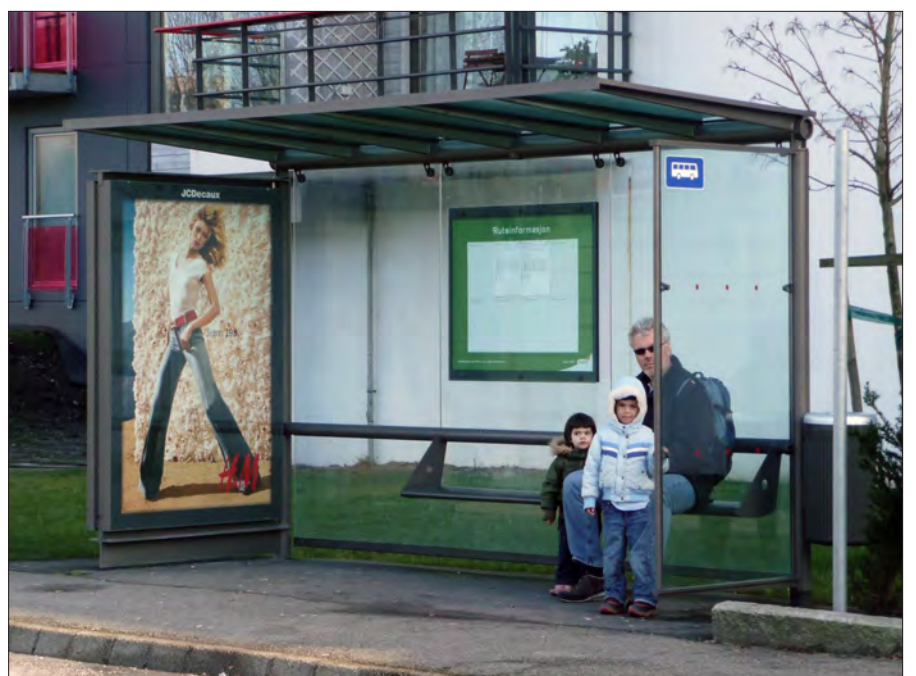
A transit stop provides an inviting and sheltered place for riders to wait for a bus.
