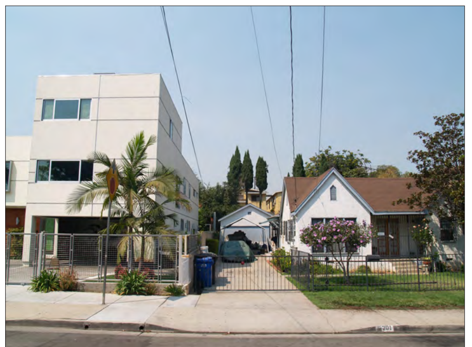
New development that is incompatible with the massing, scale, setbacks, and pedestrian-oriented disposition of buildings in historically sensitive areas.
