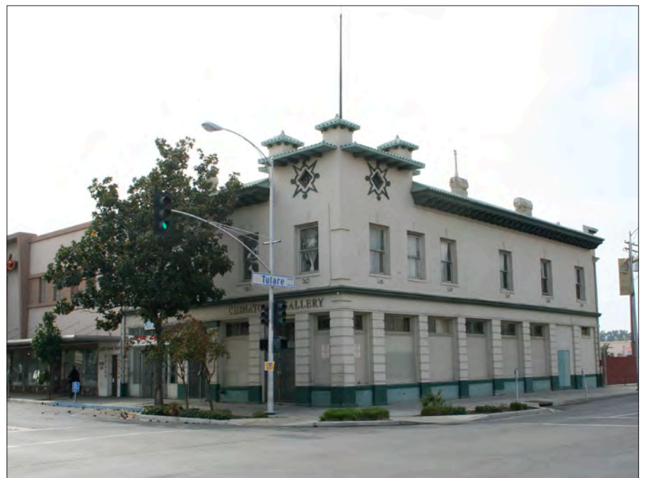
This building on the corner of F Street and Tulare Street is a source of identity and pride for Fresno residents.
