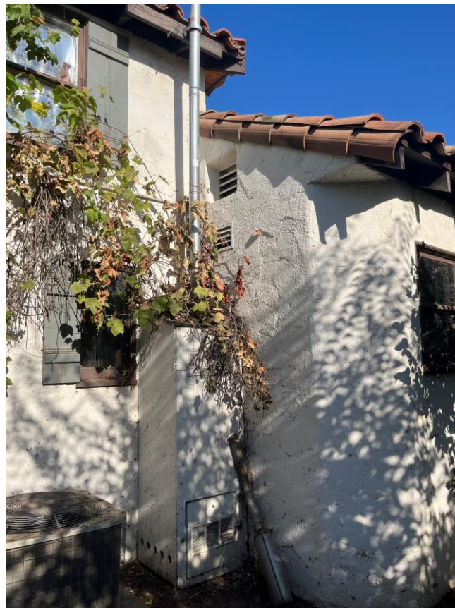
Main house, 2024, camera facing northeast
