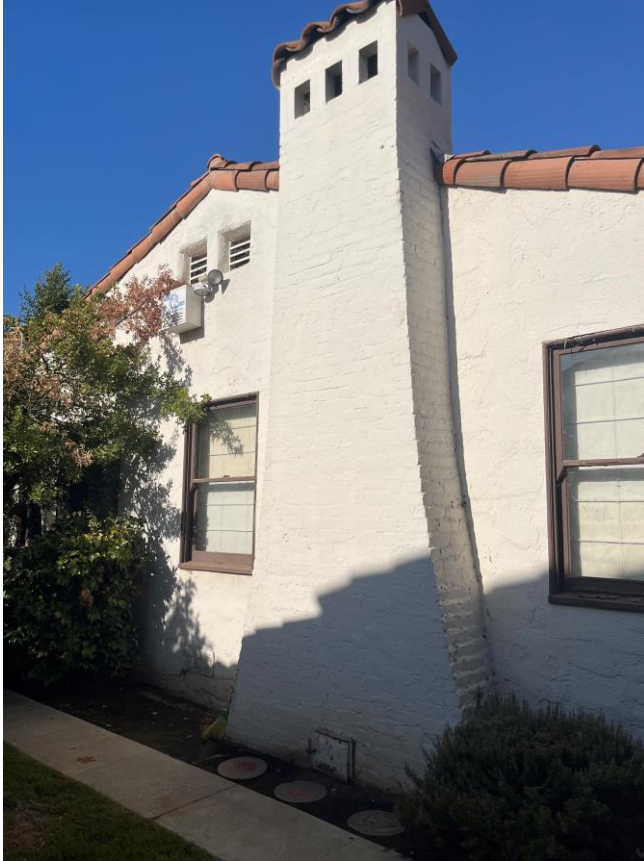
Main house, 2024, camera facing east
