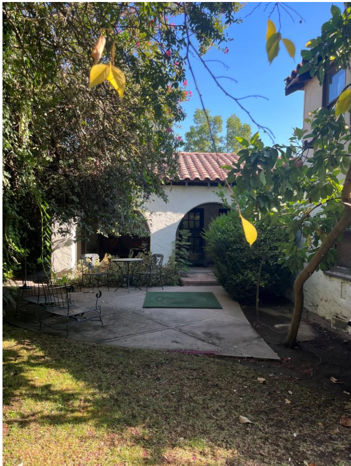
Main house, 2024, camera facing north
