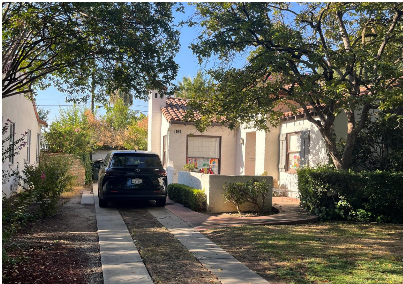
Main house, front façade, 2024, camera facing southwest
