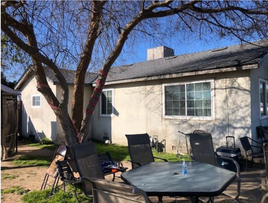
A) View looking southwest of the east facing facade of the residence. 2/28/22. Acc. #2022IMG5821
