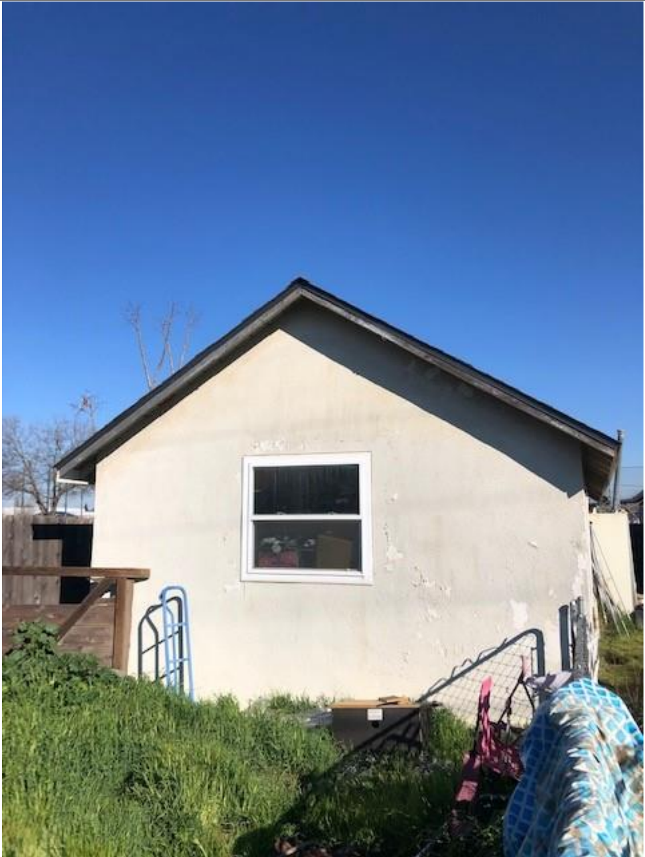
G) View looking north of the south facing façade of the detached garage. 2/28/22. Acc. #2022IMG5827
