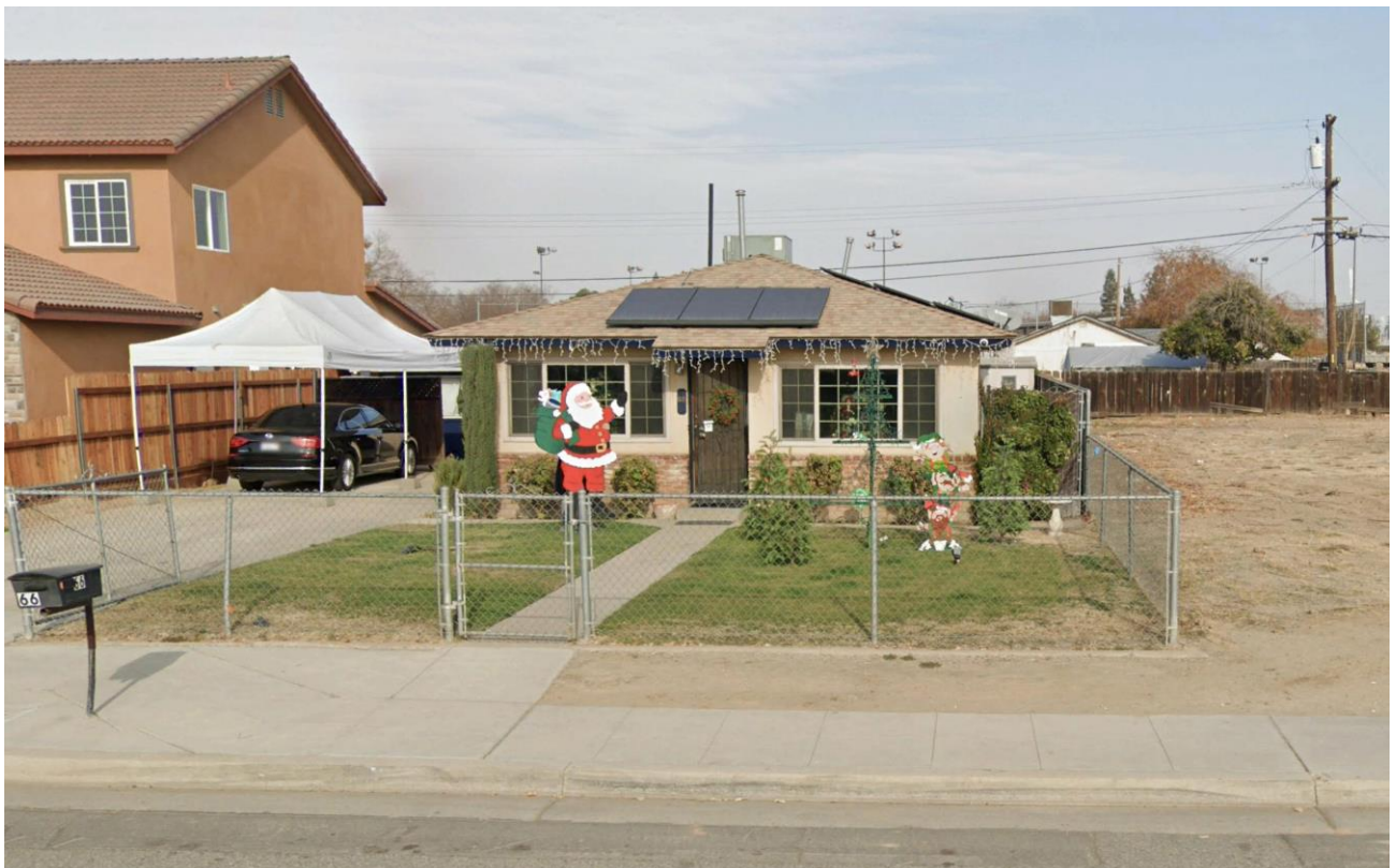
B) View looking north of the south facing façades of the garage (left), residence. 2/28/22. Acc. 2022IMG2crop
