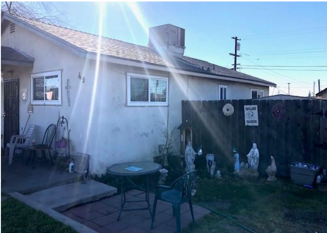
B) View looking southeast of the partial north (left) and west facing facades of the residence. 2/28/22. Acc. #2022IMG5822
