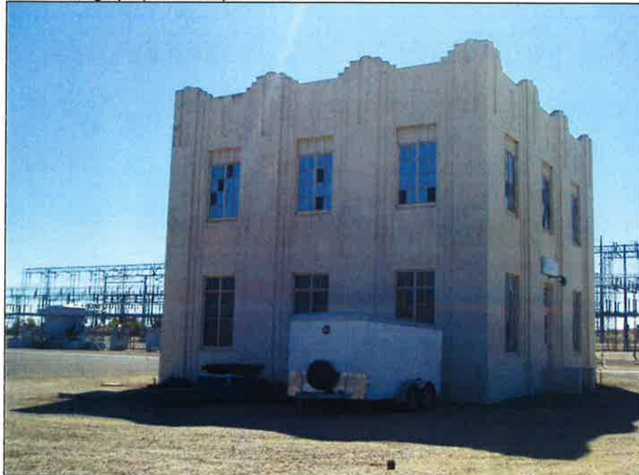
North and west elevations of Feature I, the Control Building (August 2008).
