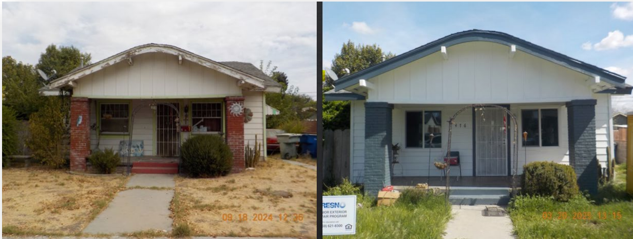
Figure 1 – Senior Exterior Repair
