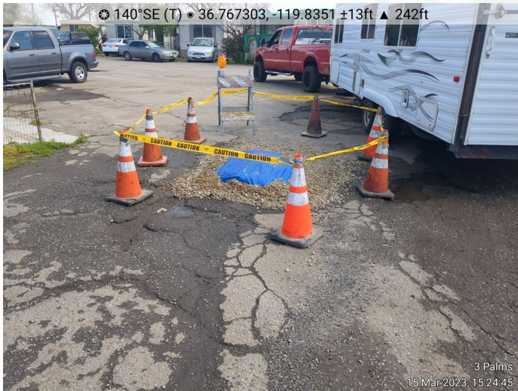
Photo 14 – Sink Hole Filled
