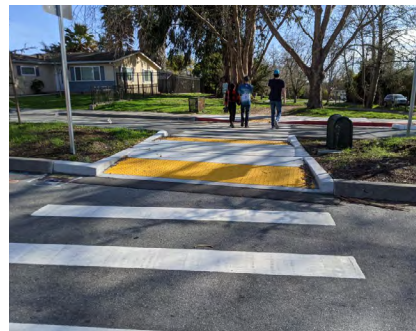
Median Refuge Island
