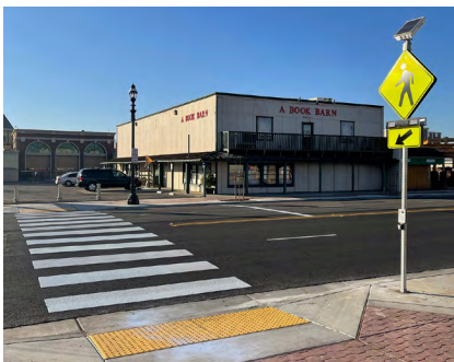
Rapid Rectangular Flashing Beacons
