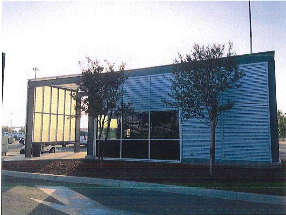
Parking Lot Office
