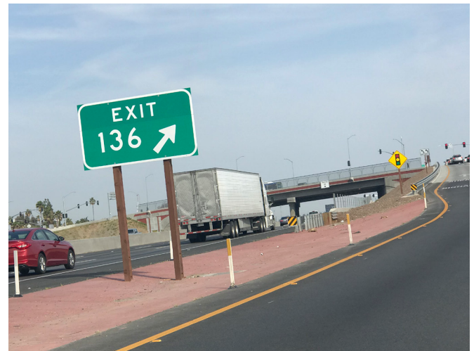
Off ramp to Clinton Ave from Highway 99.
