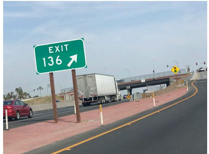
Off ramp to Clinton Ave from Highway 99.
