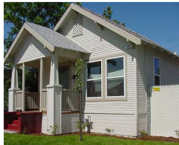
Renovated Façade on Palm Avenue Bungalow.
