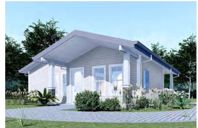
Accessory Building Design. Accessory dwelling units should have the same materials and architectural style as the primary residents, such illustrated by this Craftsman-style ADU. (Photo credit: Fresno County.)
