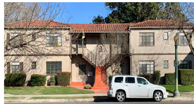
Early 20th-century apartment building with covered entry and varied massing
