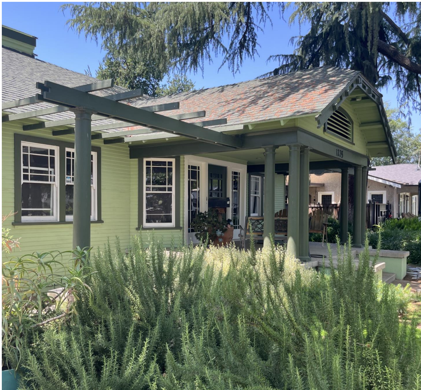
Main house, front façade, 2024, camera facing northwest
