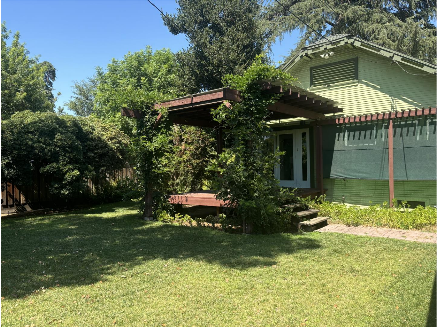
Main house, rear façade, 2024, camera facing northeast
