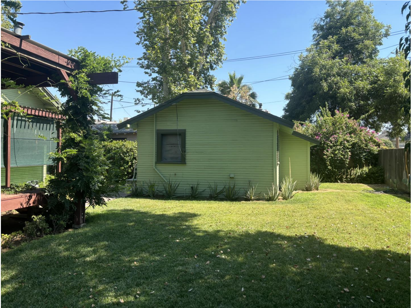
Garage, north façade, 2024, camera facing south
