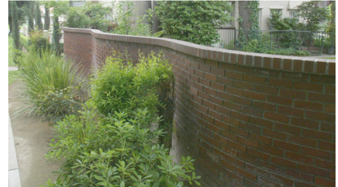
Rear Yard Fence. This corner lot rear yard fence is tastefully done to complement the residence. Notice the use of the landscaping along the sidewalk side of the fence and how it softens the appearance.
