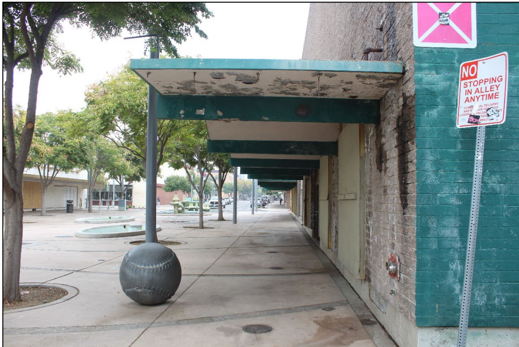
Figure 10. Detail of the cantilevered concrete canopy on the north façade of the building, facing northeast (Stantec, 2025).
