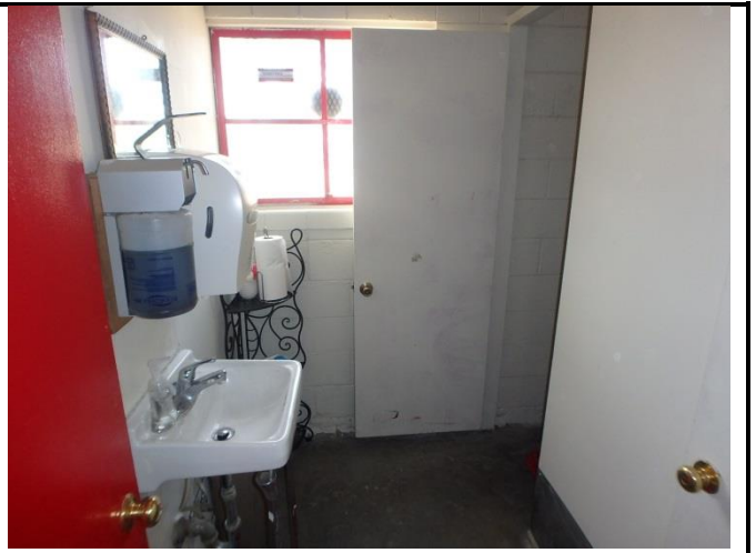
Photo 8: View of the restroom inside the food storage building
