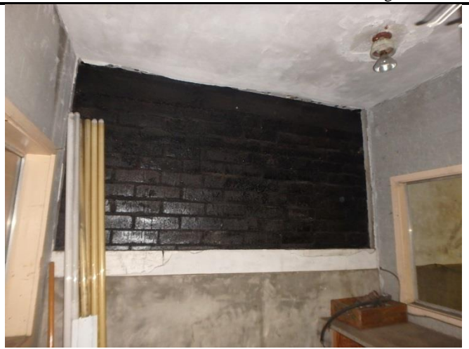
Photo 4: View of the office in storage room 2
