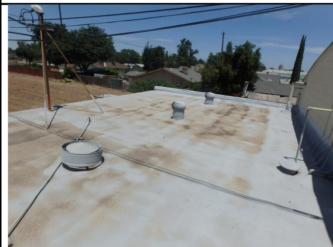
Photo 11: View of the food storage building roof
