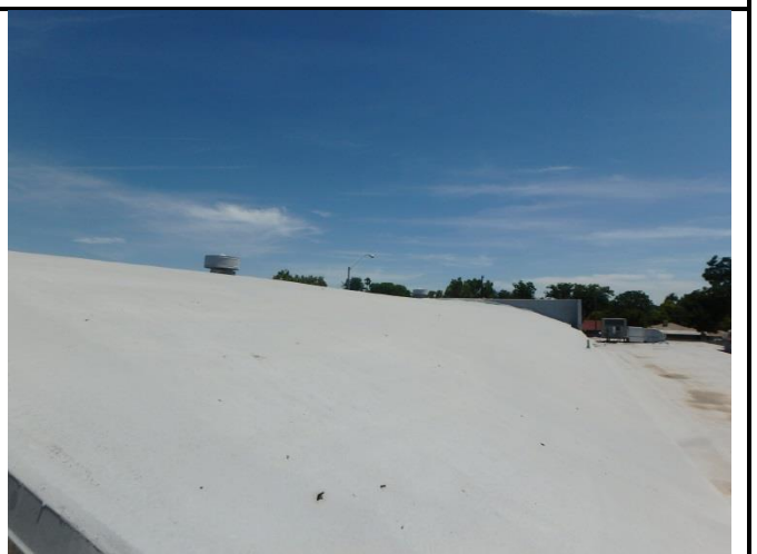
Photo 12: View of the main roof
