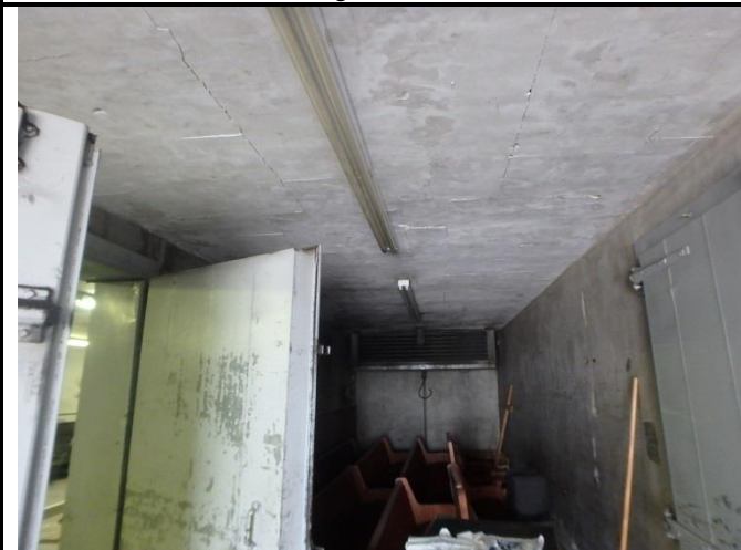
Photo 5: View of the hallway between storage room 1 and 2
