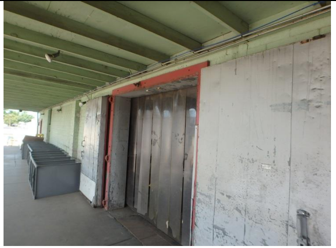
Photo 2: View of the south wall of the building
