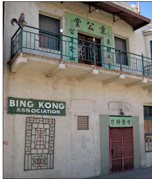
Bing Kong Association Building (1900)
