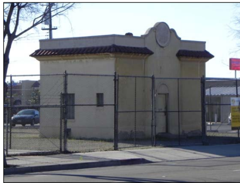
G Street Substation (c. 1920)
